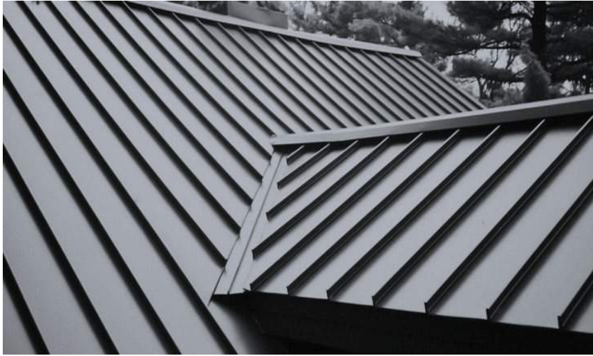
Standing Seam Metal Roof
