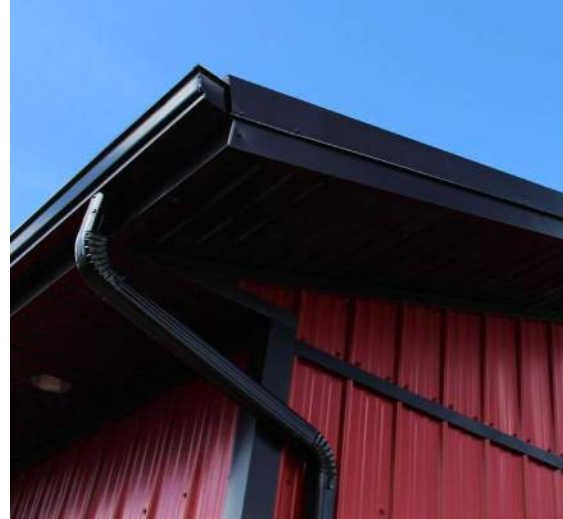
Exterior Steel + Downspouts and coping Color
