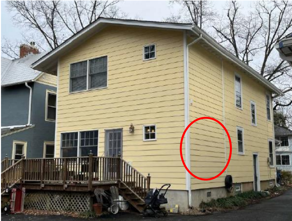
Figure 3: Left elevation with the approximate location of the approved window circled in red.
