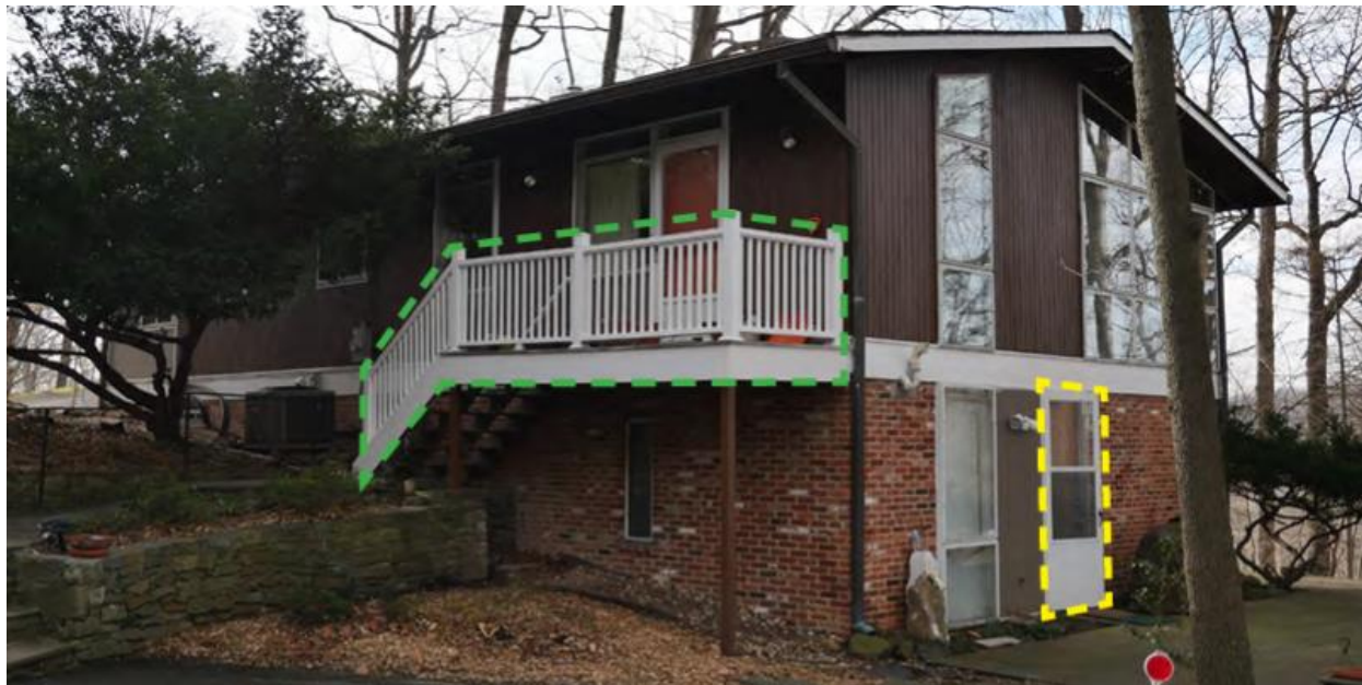
Figure 2: Image from the northeast of the subject house showing the replacement exterior stairs (in green) and the added side door (in yellow).
