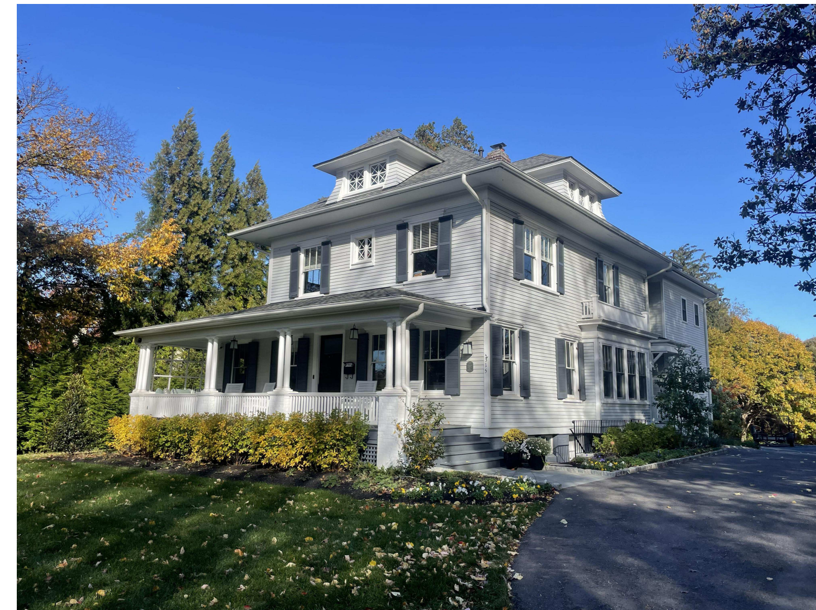
FRONT RIGHT EXISTING VIEW
