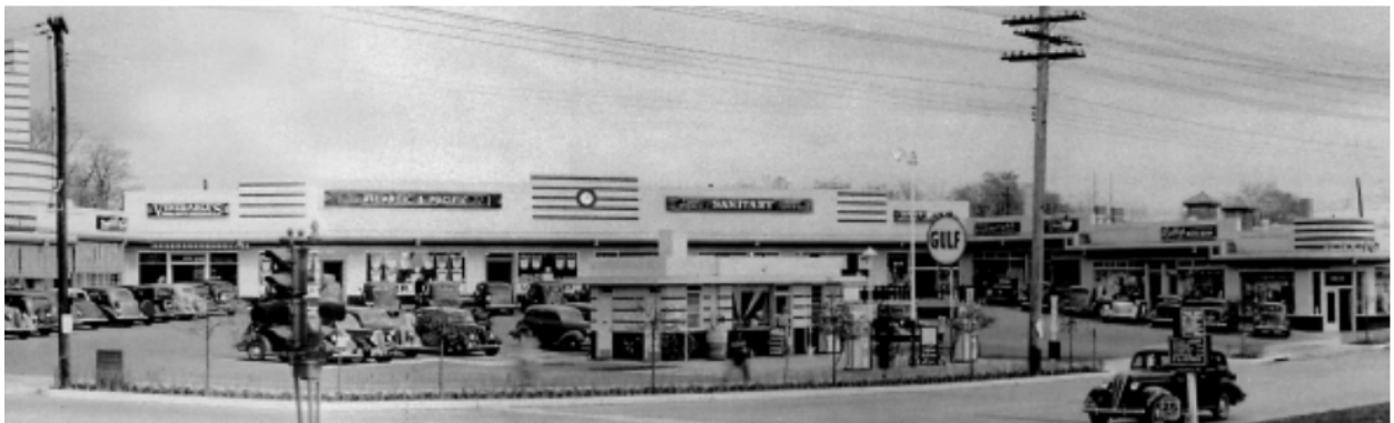
Figure 2: Silver Theatre and Shopping Center in 1938. The new tenant unit is to be located in the storefront at the far right of the photograph (The Mitchell Wolfson, Jr. Collection, The Wolfsonian-Florida International University, Miami Beach, Florida).
