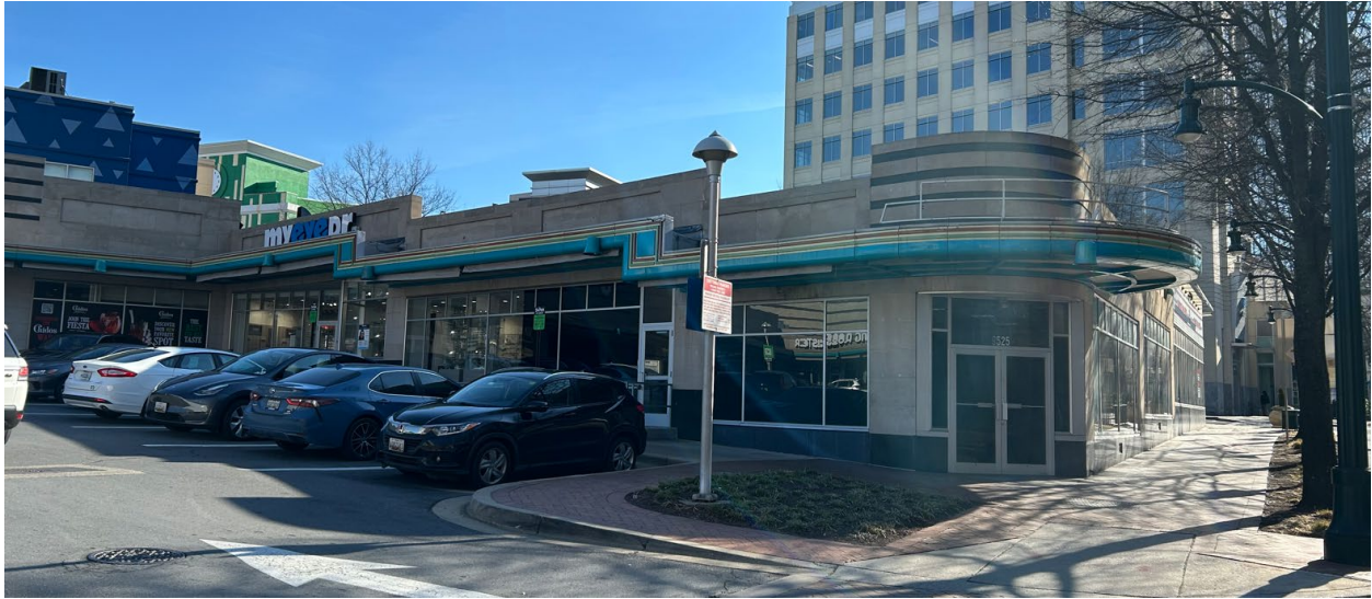
Figure 3: View of the tenant unit from the southern entrance drive (January 2026, Historic Preservation Division).
