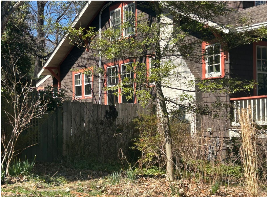
Figure 7: View of the existing fencing along the south side of the house (March 2026, Historic Preservation Division).
