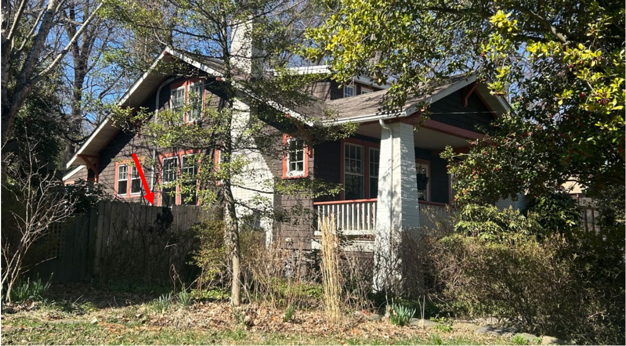
Figure 2: View of the south side of the house and the location of one section of existing fencing to be replaced. Two of the three windows proposed for replacement are located behind the fence at the foundation level (March 2026, Historic Preservation Division).
