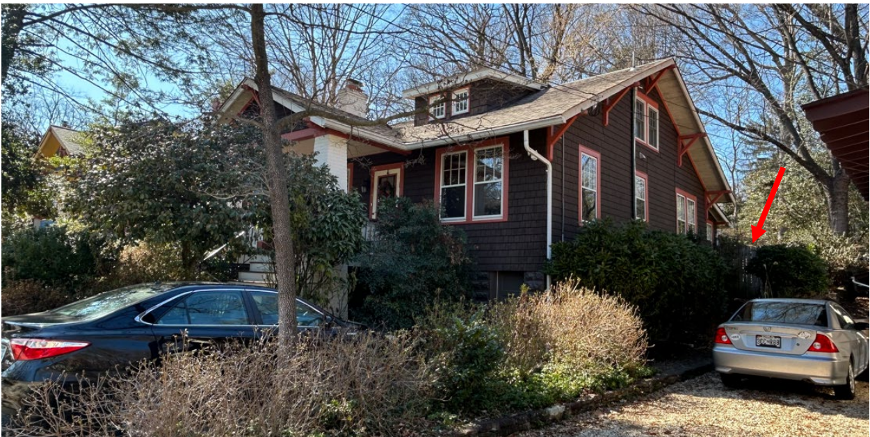
Figure 3: View of the north side of the house and the location of the other section of existing fencing to be replaced. One of the three windows proposed for replacement is located along this elevation behind existing shrubbery (March 2026, Historic Preservation Division).
