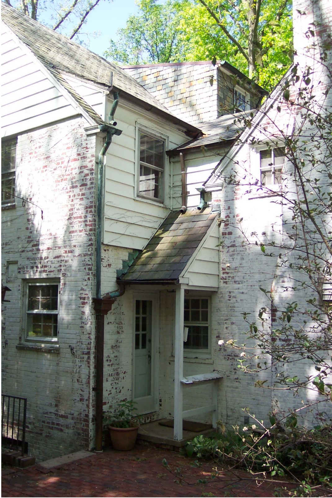
5605 York Lane photo of existing covered rear stoop (image #2)
