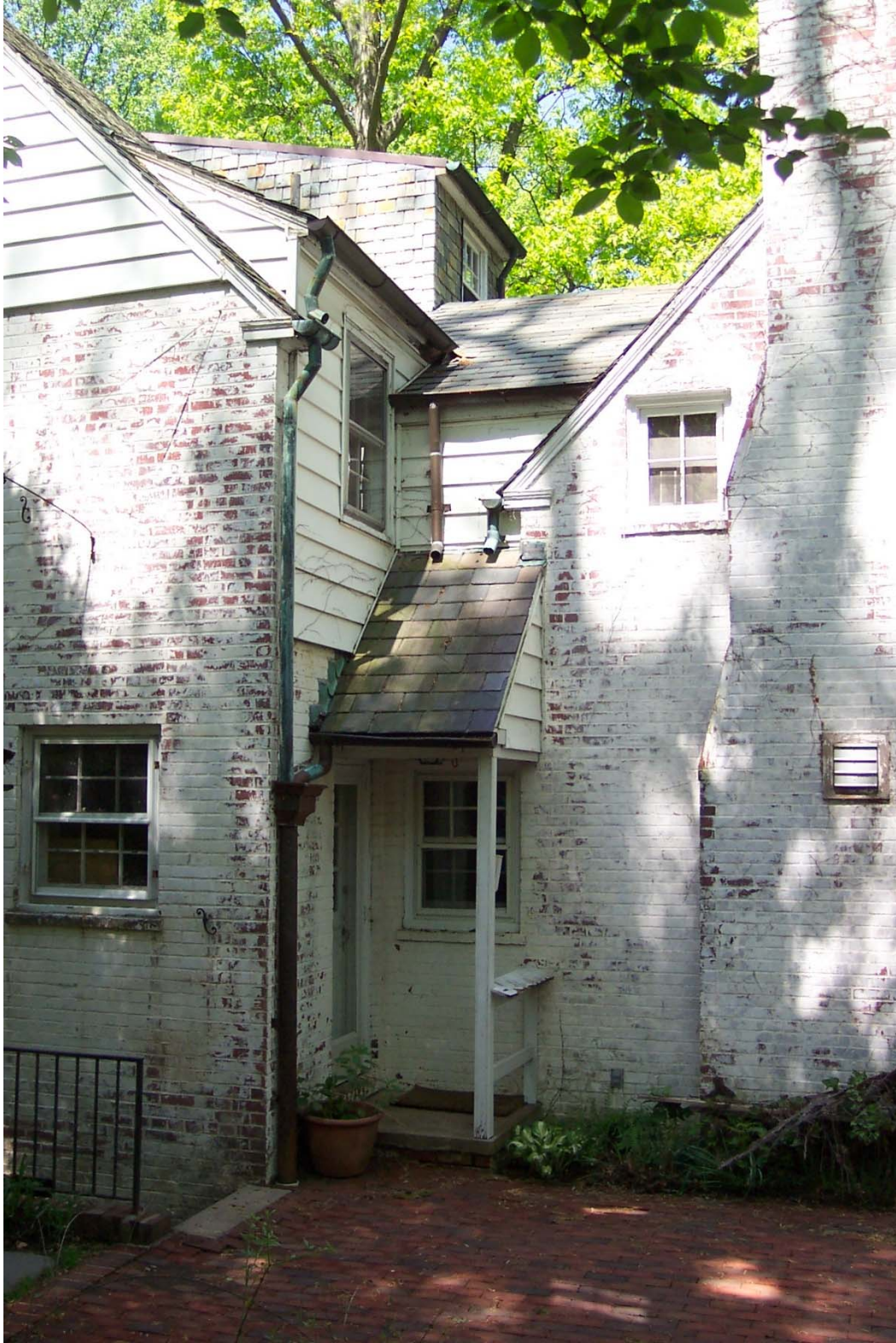
5605 York Lane photo of existing covered rear stoop (image #1)
