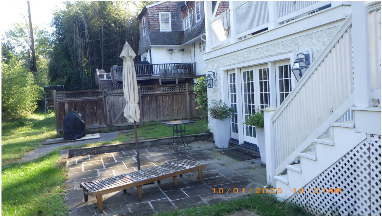
Figure 3. Existing stone patio and stairs to be removed to expand covered porch to proposed screened porch.
