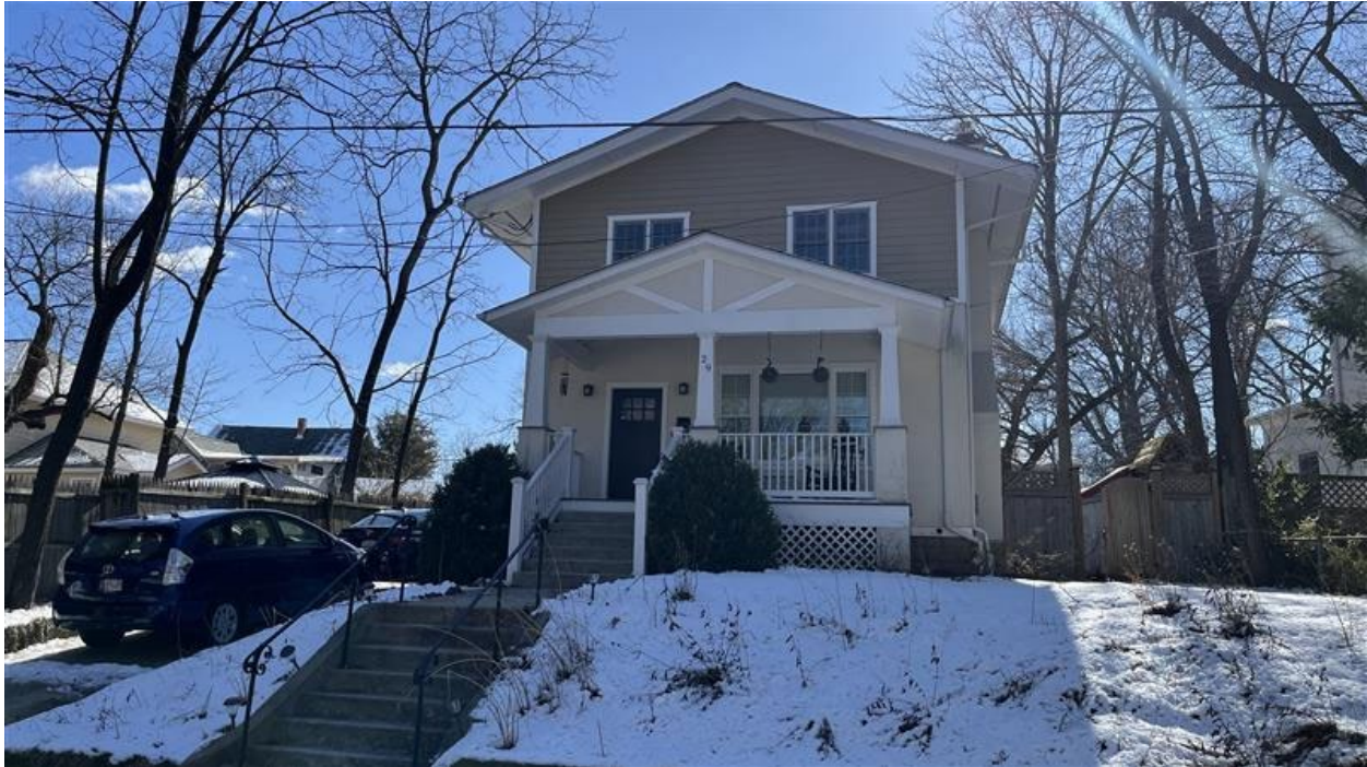
Figure 2: View of subject property along Holt Place.
