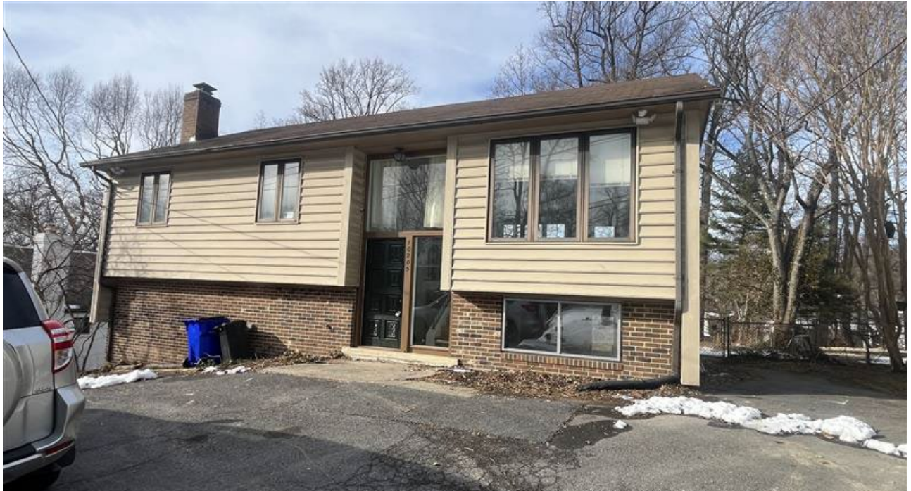
Figure 3: Facade of subject property from Capitol View Avenue.
