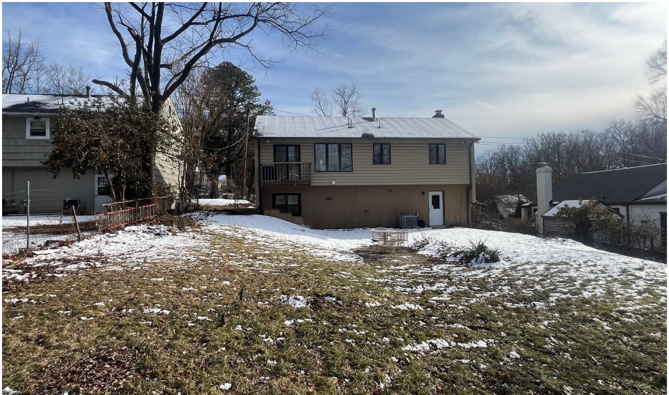
Figure 4: Rear view of the subject property.
