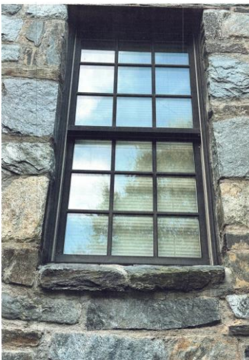
Figure 7: Existing aluminum-clad windows (left) and specifications for proposed aluminum-clad Trimline sash kit (right).
