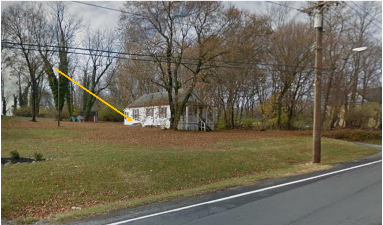
Figure 4: View of subject property from the right-of-way along Frederick Road. The location of the unit is notated with a yellow arrow.
