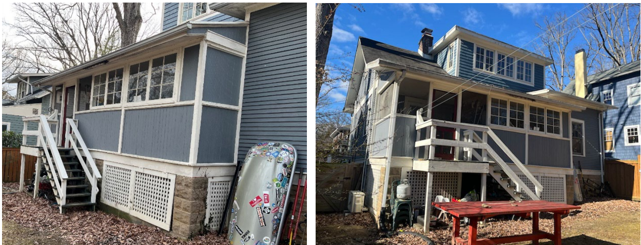
Figure 3: View of the rear porch.
