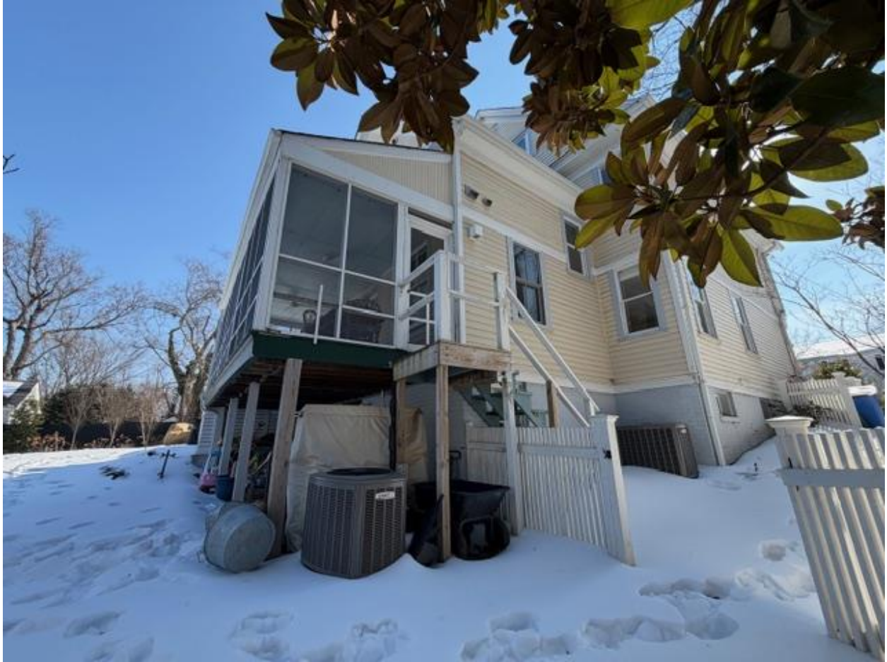
Northwest view (rear/west façade):
