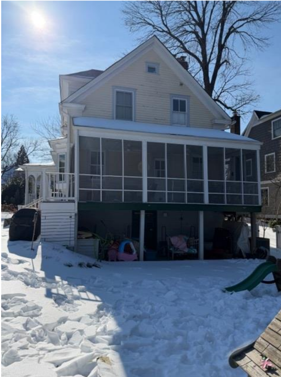
North View (rear façade):
