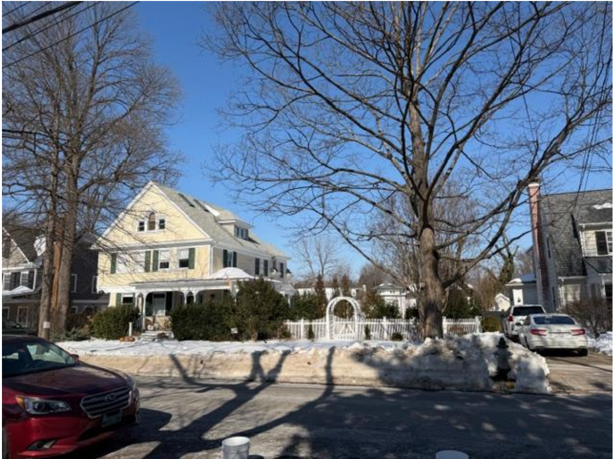
South View (front façade):
