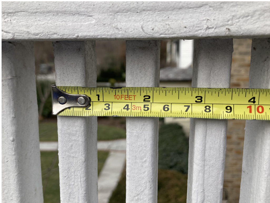
1 Exist. Baluster Dtl., Porch Roof
