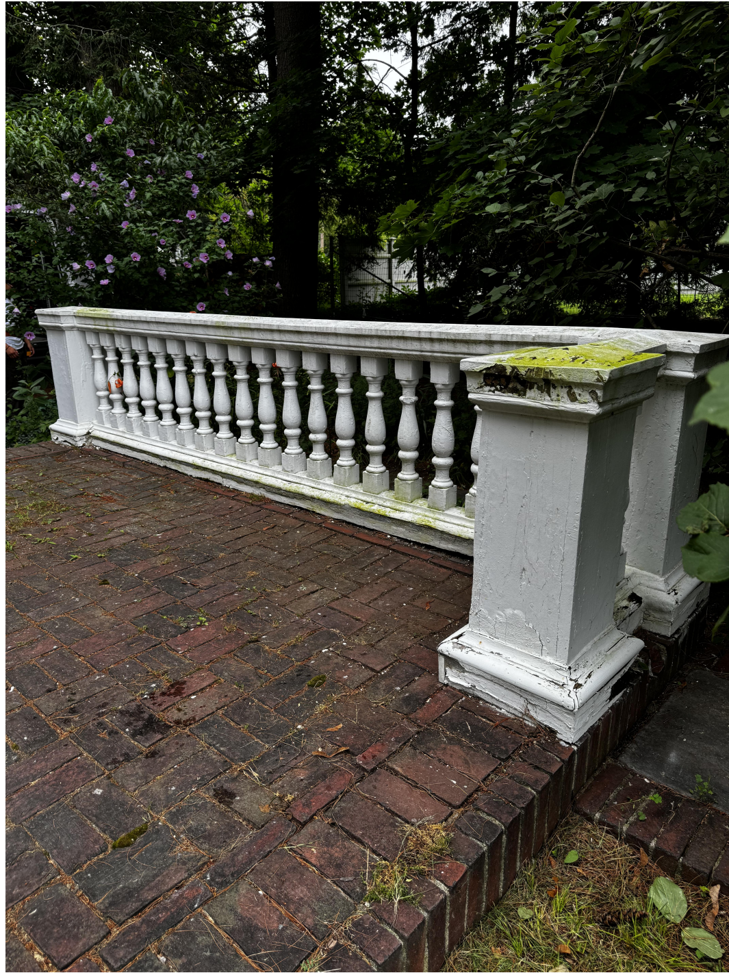
Example of a historical railing replicated using the Nautilus custom milled cellular PVC product.
