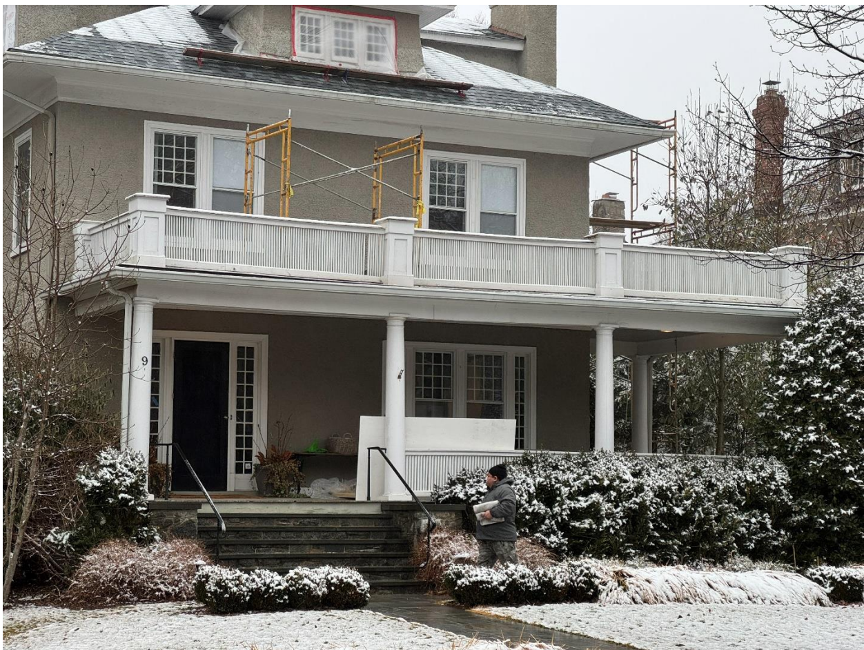
Figure 2: Front elevation of the subject property, the bottom balusters are noticeably wider.
