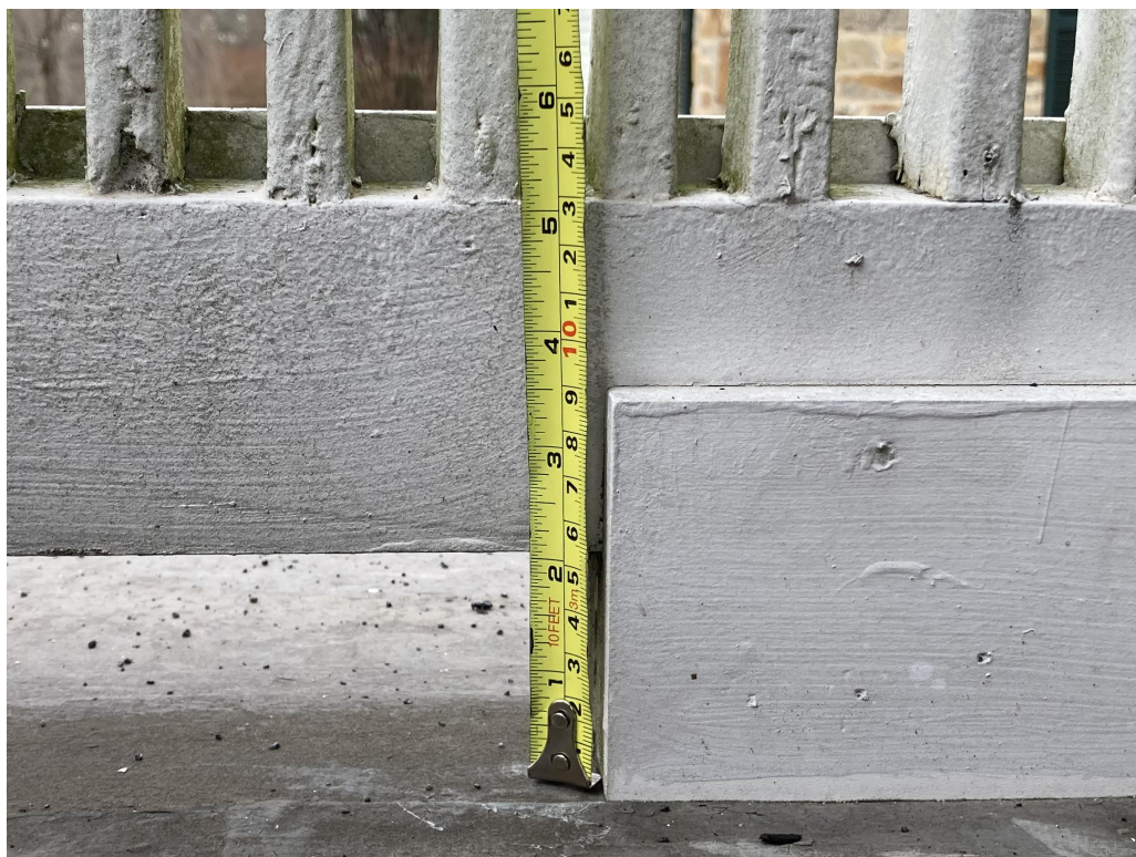
3 Exist. Btm. Rail Dtl., Porch Roof
