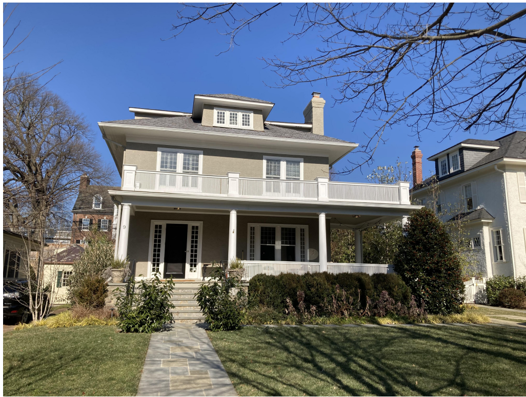
1 Front (South) View
