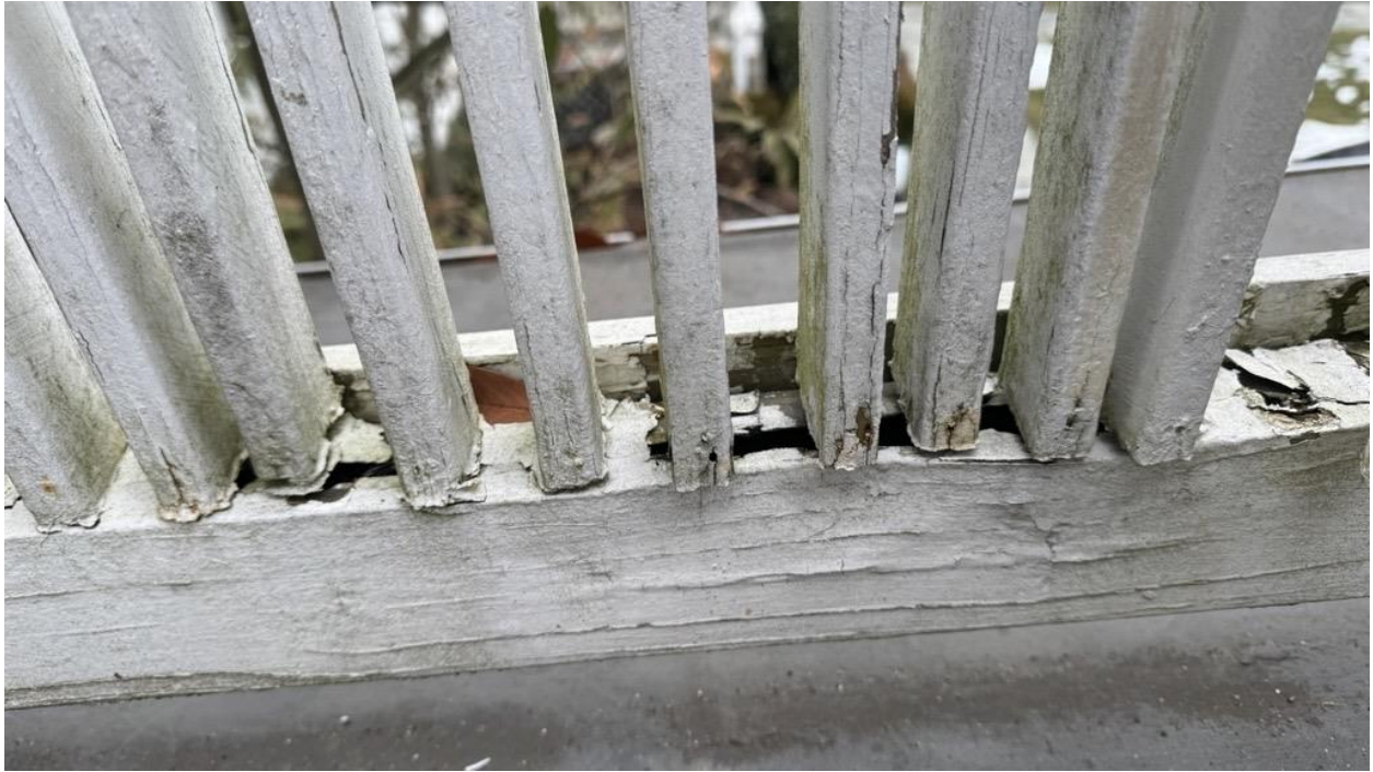
Figure 4: Detail of the existing railing condition.
