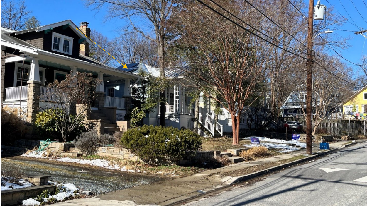
Figure 8: View of roof from right-of-way. The location of panels is notated with a yellow arrow.
