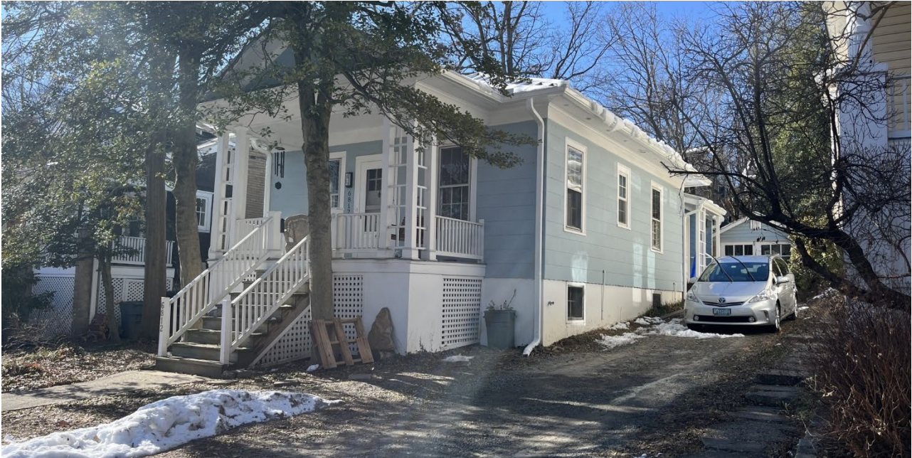
Figure 2: Subject property from the right-of-way along Westmoreland Avenue (c. 1992).
