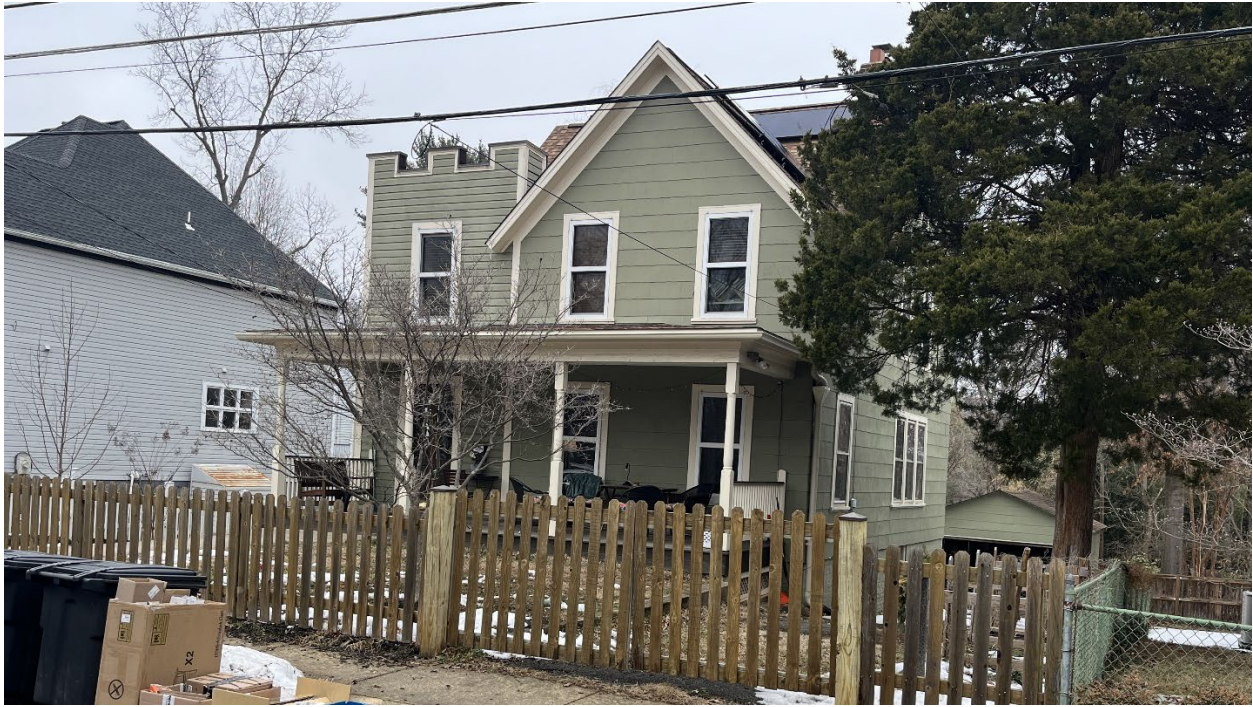
Figure 2: View of subject property along Takoma Avenue.
