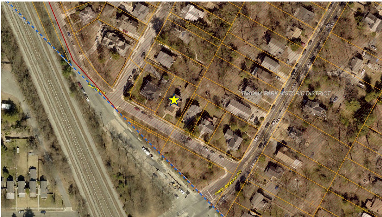
Figure 1: The subject property at 7307 Takoma Avenue in the Takoma Park Historic District is indicated with a star.
