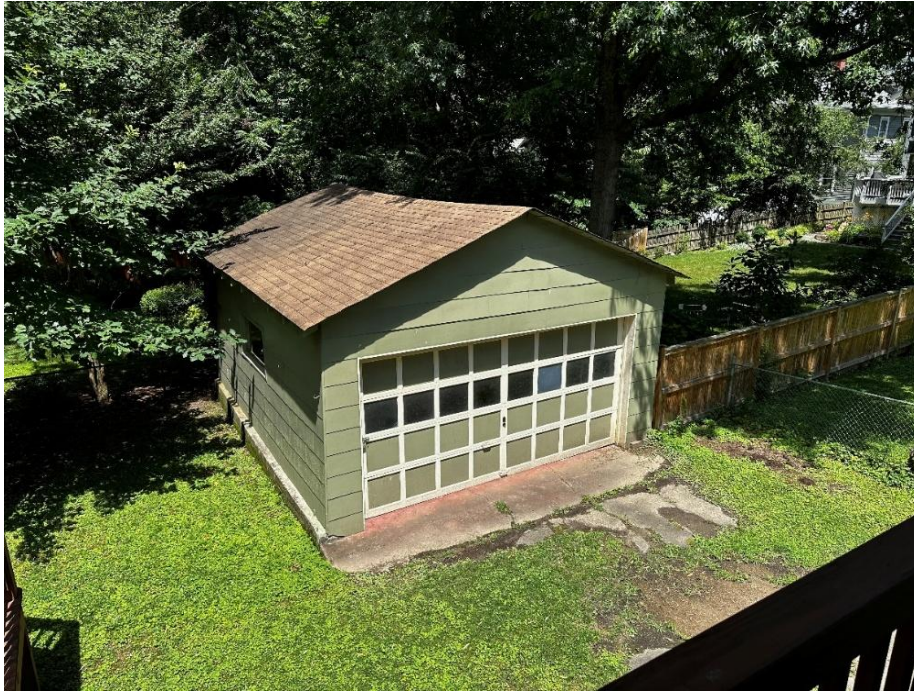
Figure 4 - Existing Garage view from Southwest
