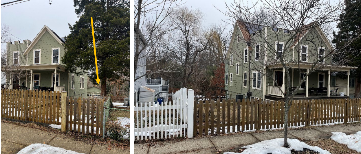
Figure 8: View of the subject property from the right-of-way along Takoma Avenue. The location of the existing garage is identified with a yellow arrow.
