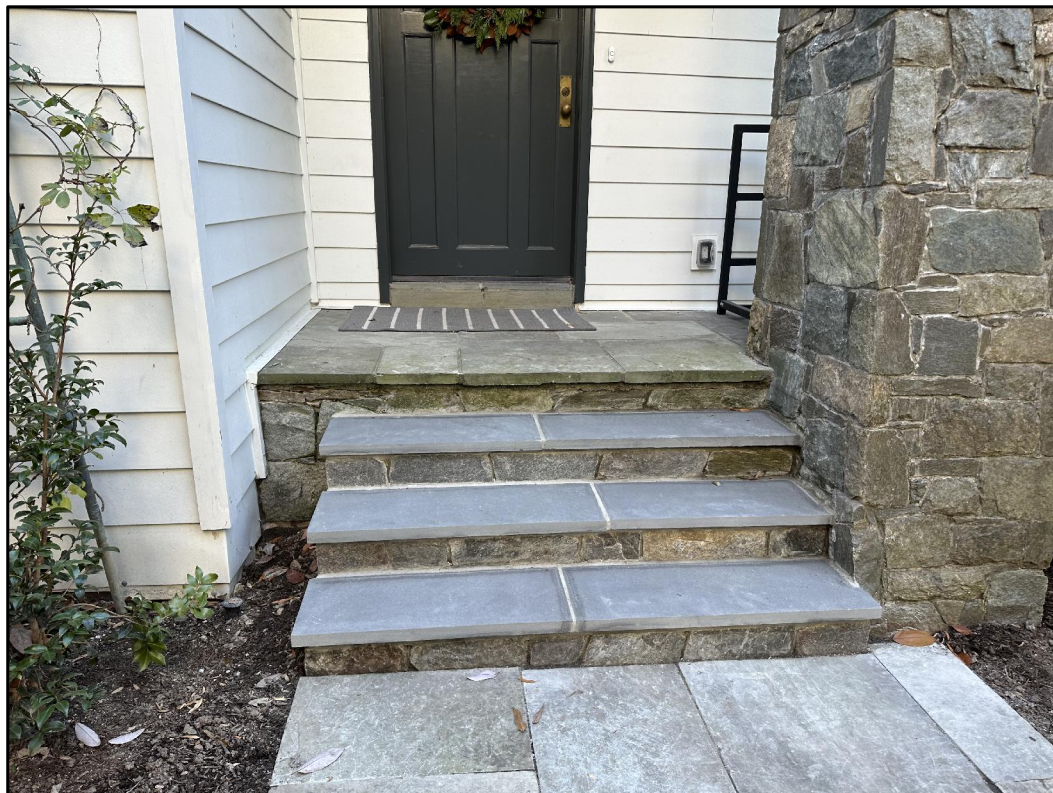
Bluestone Tread Stairs with Stone Risers
