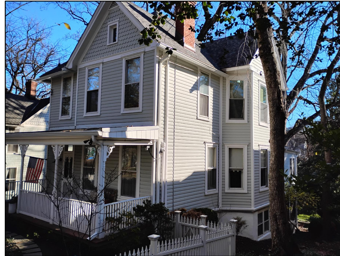
View of Southern Existing Side-yard of Residence (November, 2025)
