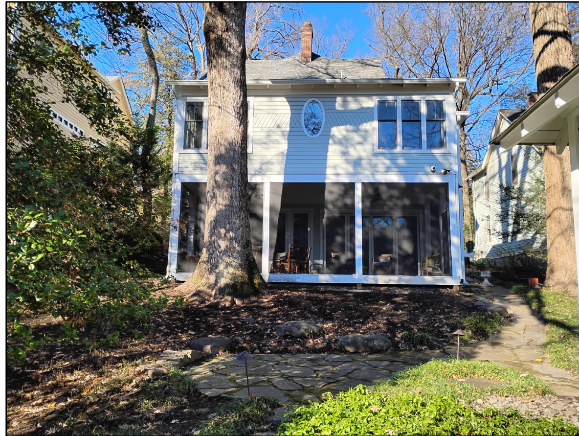
View of Existing Rear of Residence (November, 2025)
