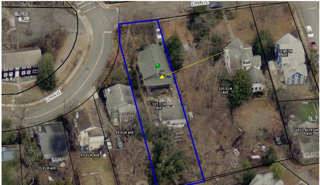
Figure 7: Aerial View of subject property, with non-historic addition notated with a yellow arrow.
