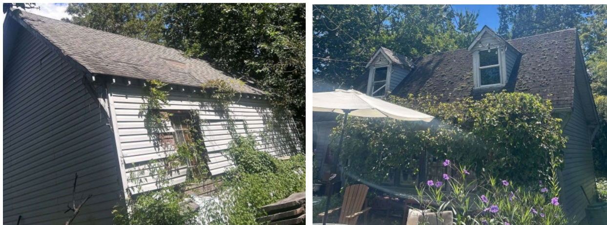
Figure 6: Photos of the accessory structure (2025).
