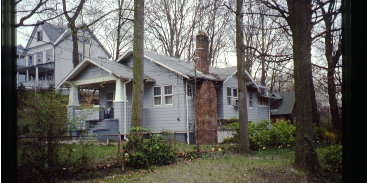
Figure 2: Subject property from the right-of-way along Elm Avenue (c. 1992).
