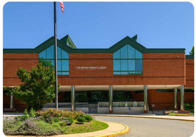
Long Branch Community Recreation Center
