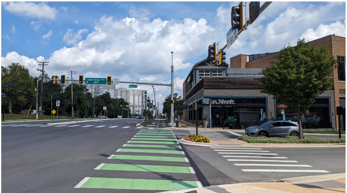
Protected Bike lanes at Rose Avenue
