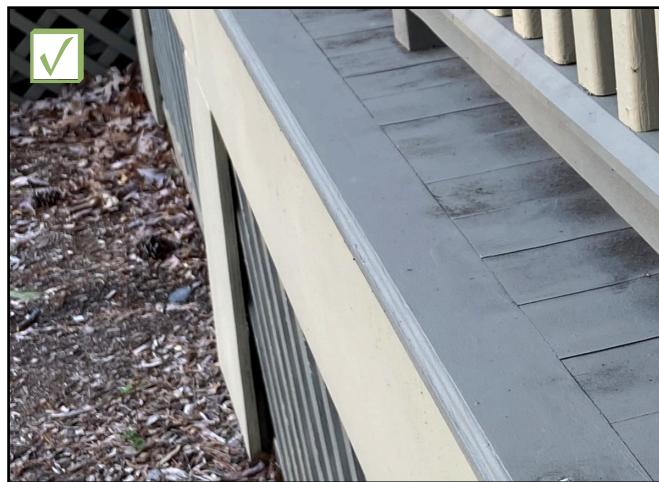
*Recommended: Boards with edges that do not replicate the appearance of wood should be finished with a board to conceal the ends.*
