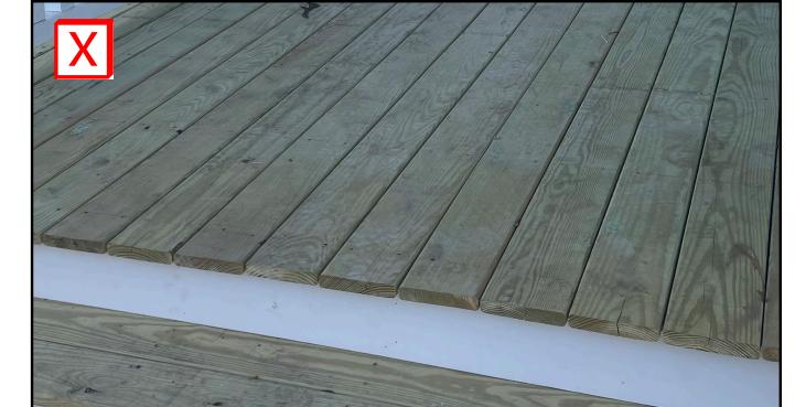
Not recommended: Standard wood boards without a tongue and groove profile are not historically appropriate for porches.
