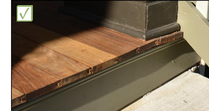
Recommended: "Tongue and groove" boards are historically accurate and should be installed on historic houses.
