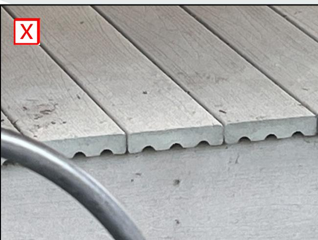
*Not recommended: The edge does not have the same texture as a solid wood board and is both exposed and unpainted.*
