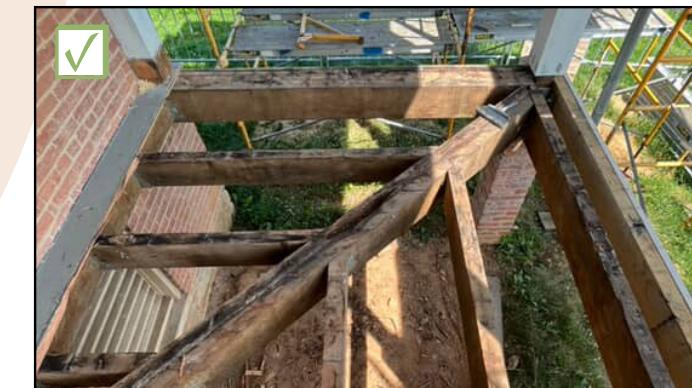
Recommended: Boards installed perpendicular to the wall with a finished edge are historically appropriate.
