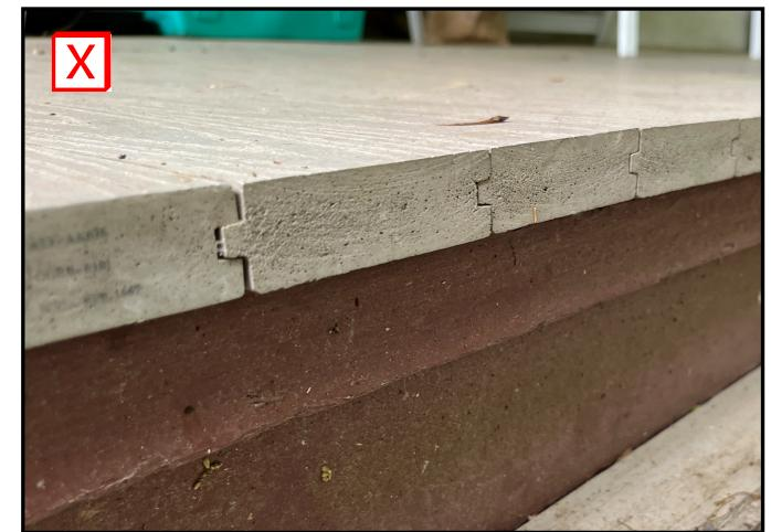
*Not recommended: The edge does not have the same texture as a solid wood board and is not finished with a concealing board.*
