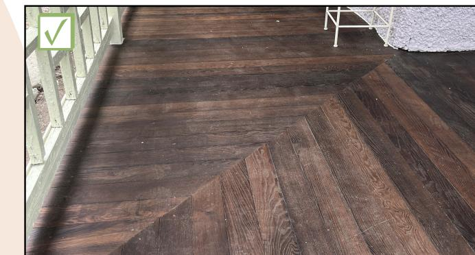
Not recommended: Standard wood boards without a tongue and groove profile are not historically appropriate for porches.
