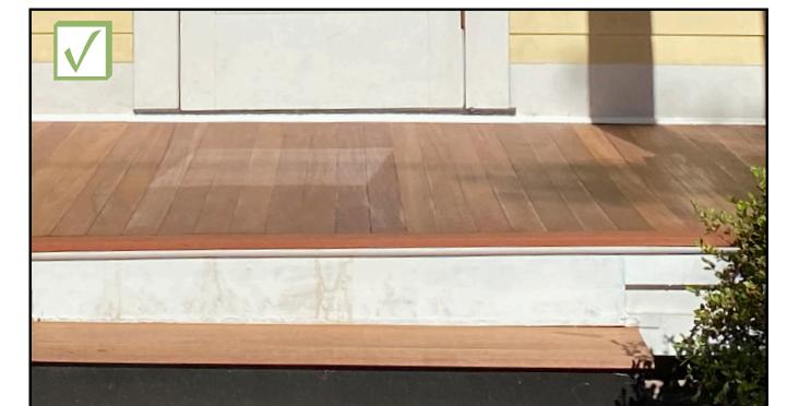
Recommended: Boards installed perpendicular to the wall with a finished edge are historically appropriate.
