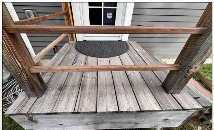
*Caption: Thermally modified wood on a deck, two years after installation.*
