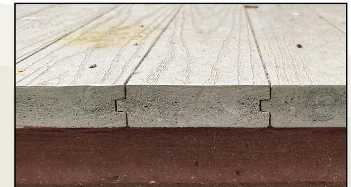
*Caption: PVC and composite decking often have a manufactured edge that does not replicate the look of wood. These edges should be covered.*
