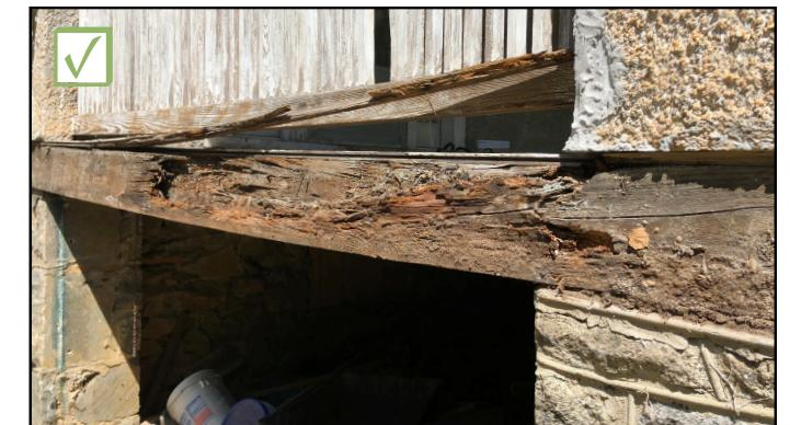
Recommended: Damaged wood should be replaced as needed.
