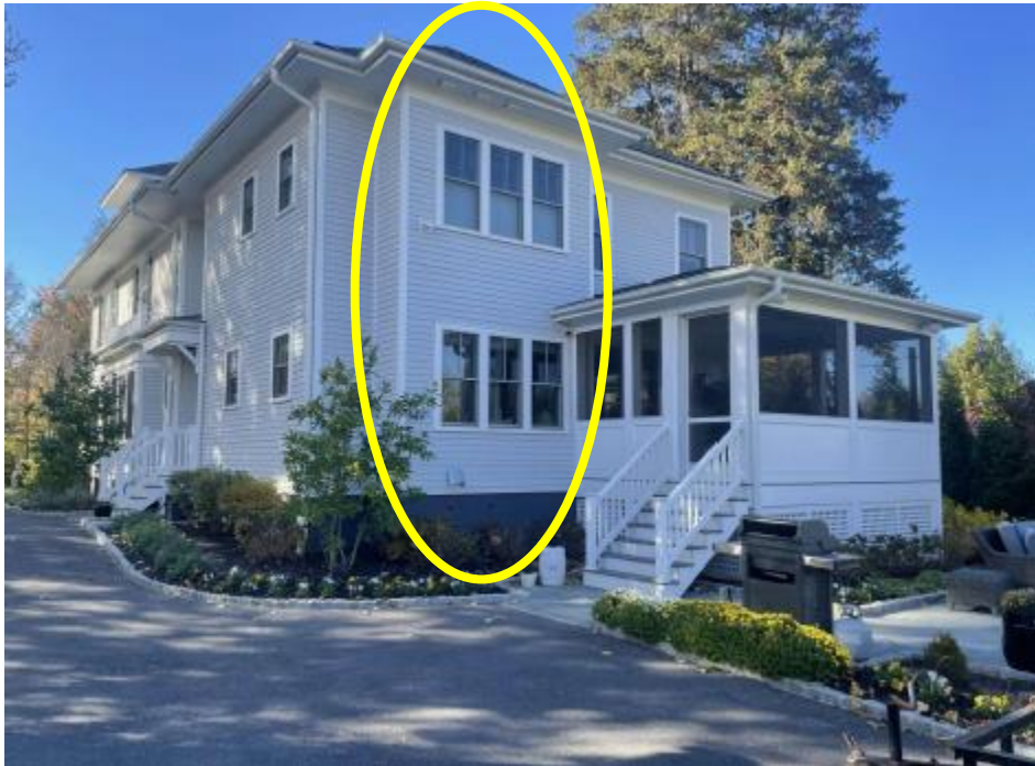
Figure 5: The projecting bay, circled in yellow, will extend approximately 7' (seven feet) further to the rear.
