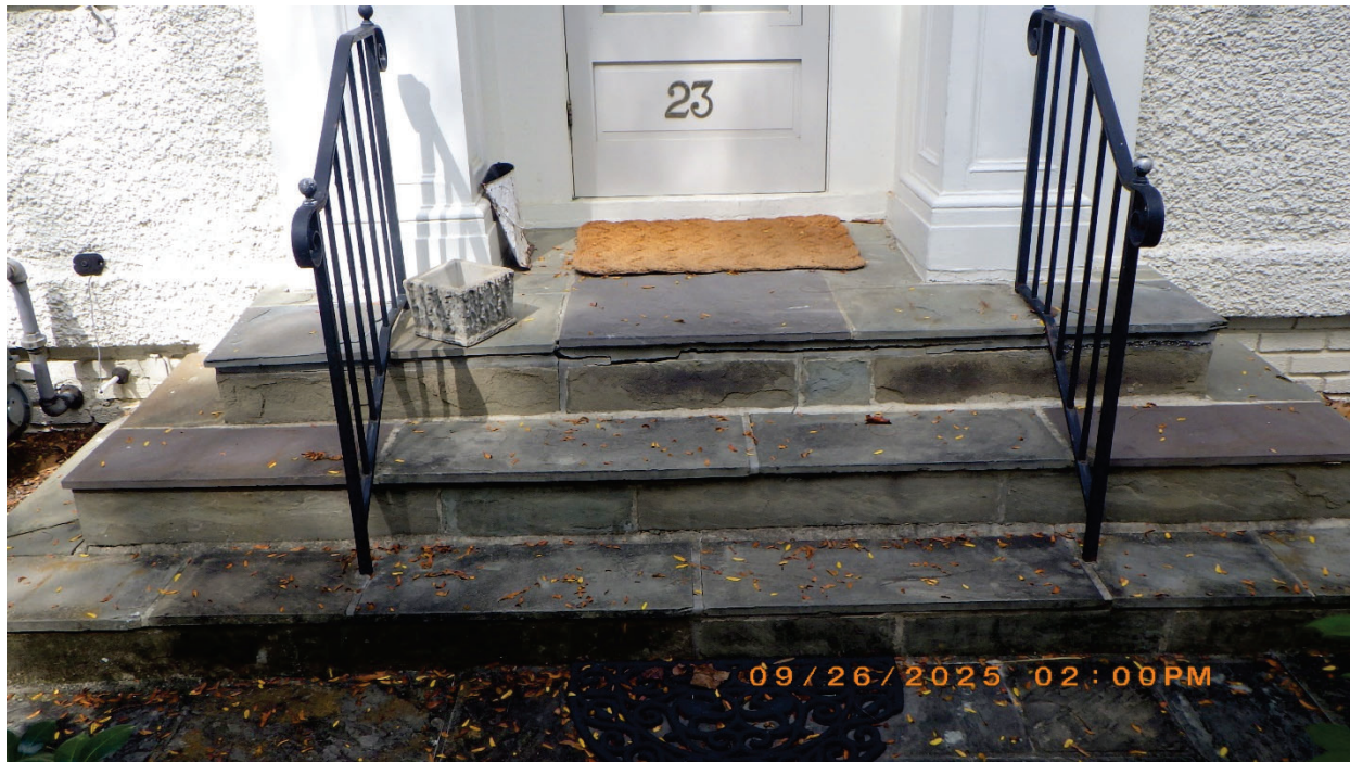
Figure 2. Existing front portico/step to be replaced
