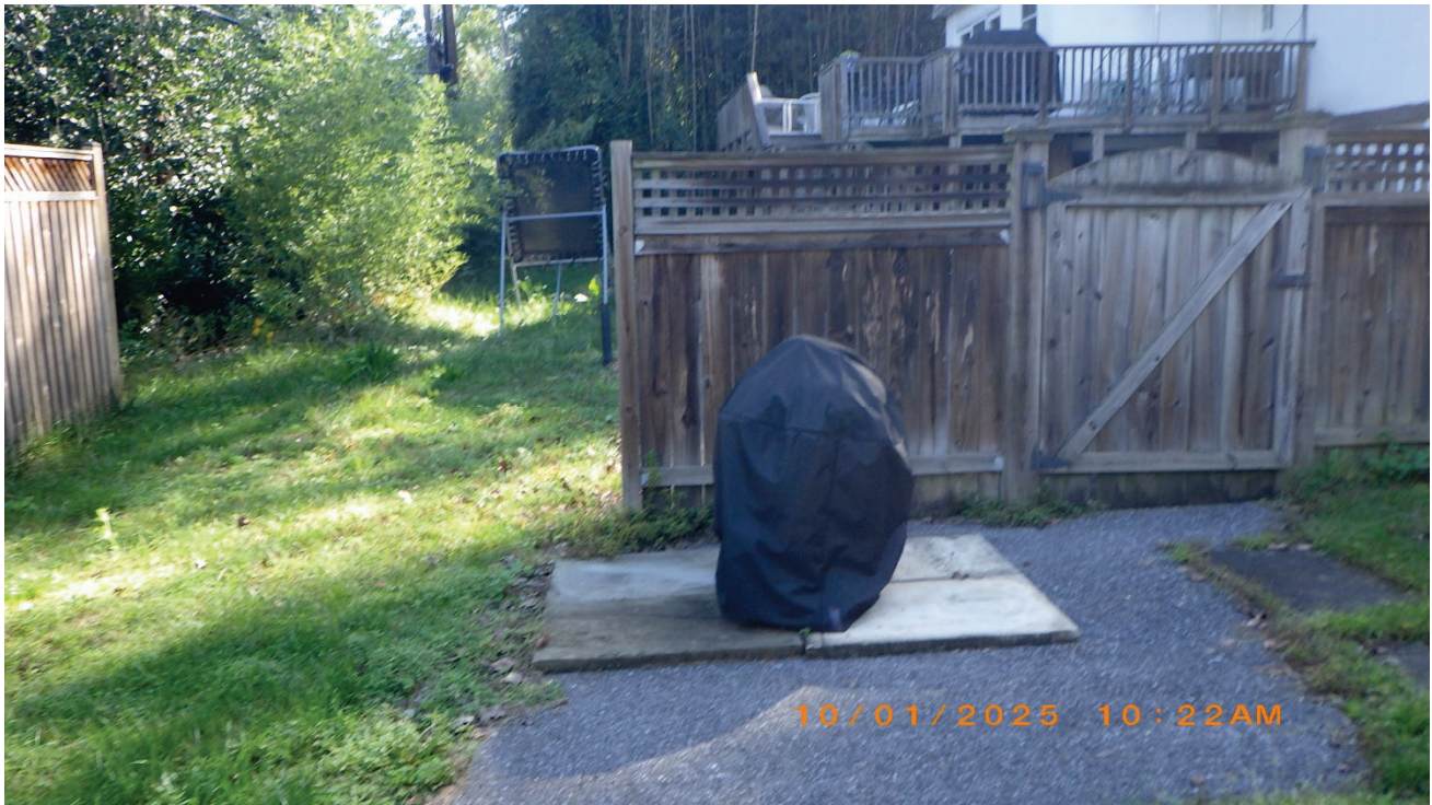
Figure 4. Existing asphalt apron to be removed.
