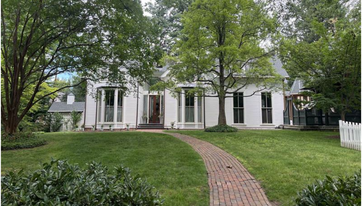
Figure 3: The façade of the subject property from West Irving Street. An addition is proposed where the gazebo is currently located.
