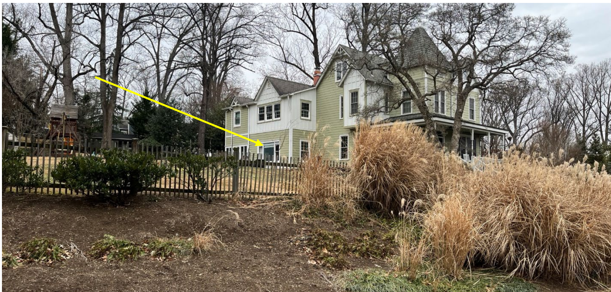
Figure 6: View of subject property from the right-of-way along Waverly Avenue. The approximate location of the deck is notated with a yellow arrow.
