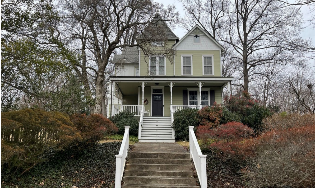
Figure 3: View of subject property from Montrose Avenue (2025)
