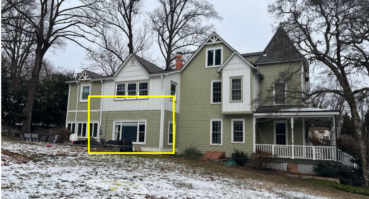
Figure 5: Side view of the subject property. The approximate location of the proposed screen porch is annotated with a yellow box.
