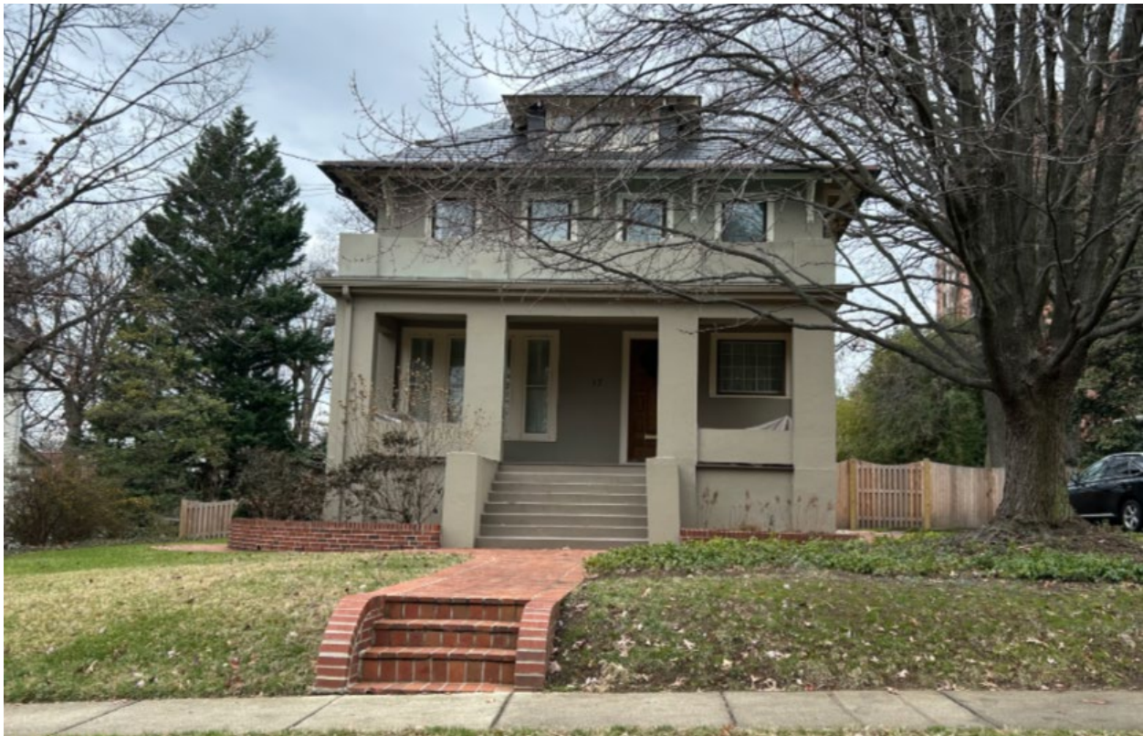
Figure 2: Front elevations of the subject property (January 2026, Historic Preservation Office).
