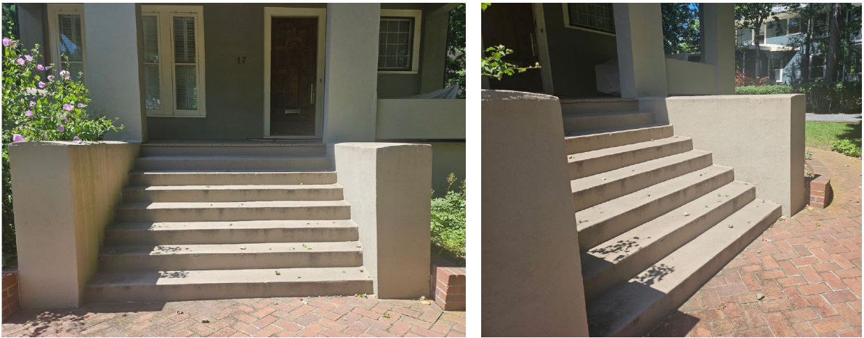
Figure 6: Existing conditions of the front steps.
