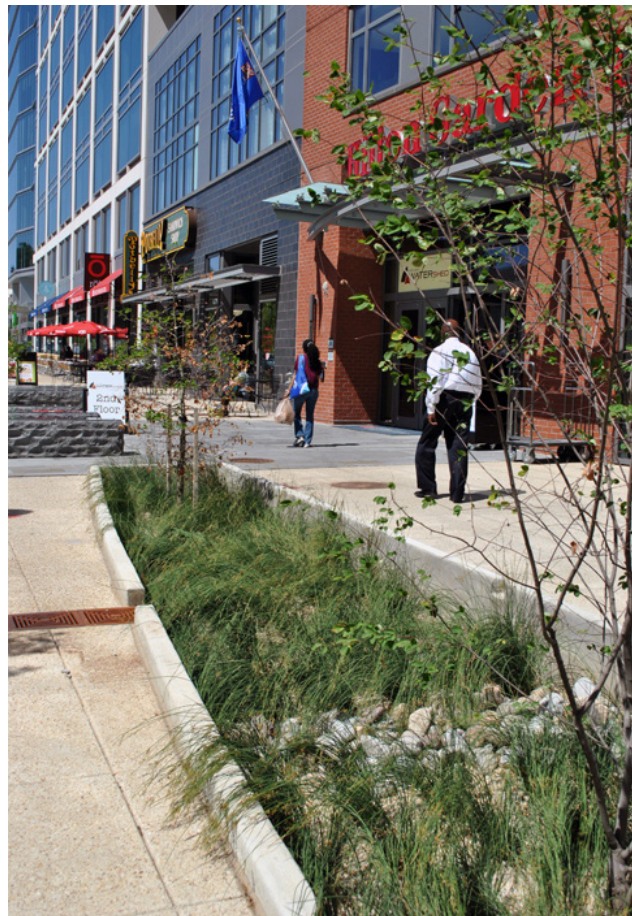
An example of stormwater management facility that is part of the streetscape design in the NOMA neighborhood in Washington, D.C.
