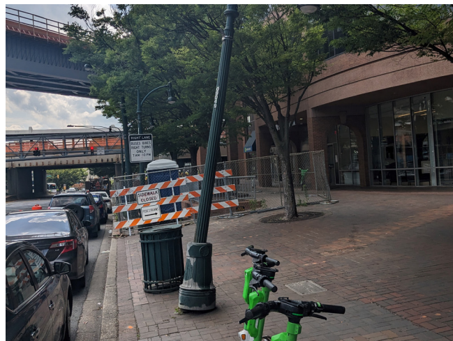
Light pole damaged by vehicle collision.
