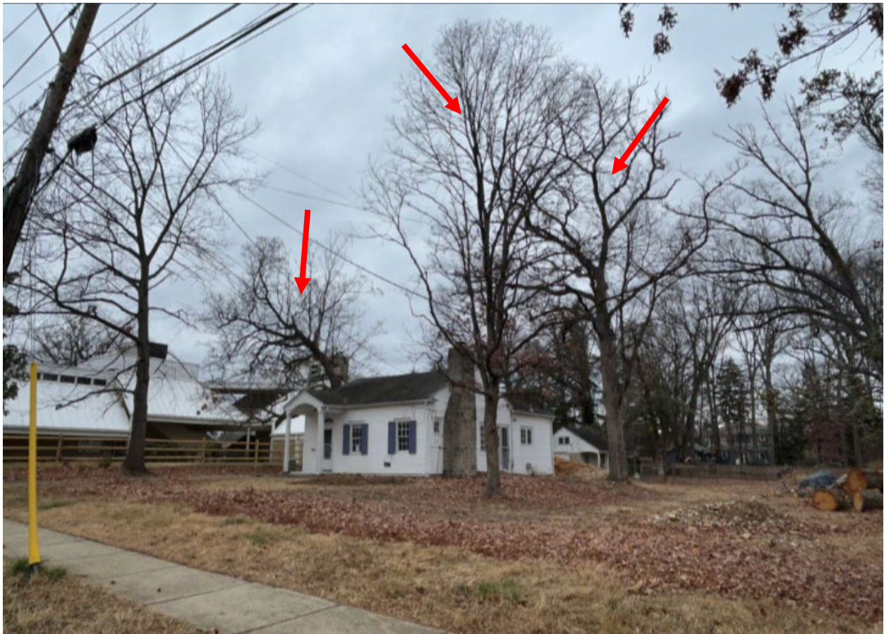
Figure 6: View of the subject property from New York Avenue. Red arrows point to the three trees proposed for removal (December 2025, Historic Preservation Division).
