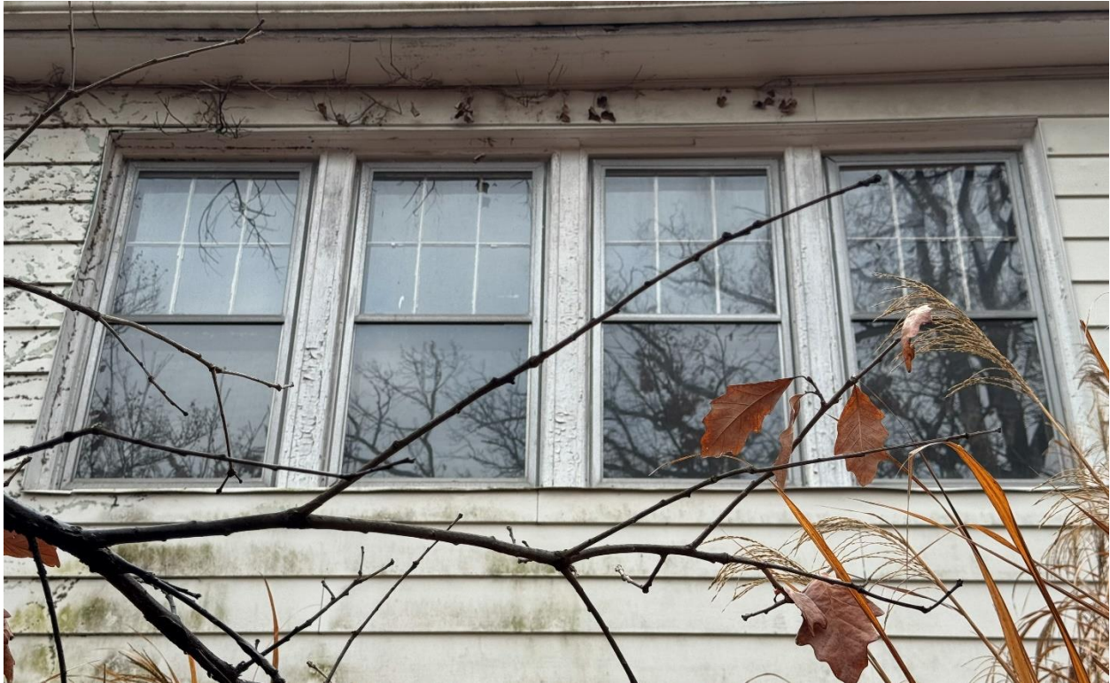
Figure 4: Ganged window in the east elevation of the sun porch.
