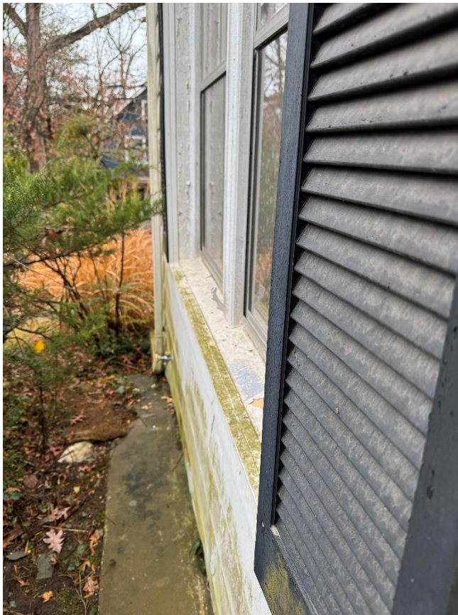
Figure 2: Detail of the existing sill on the north elevation.
