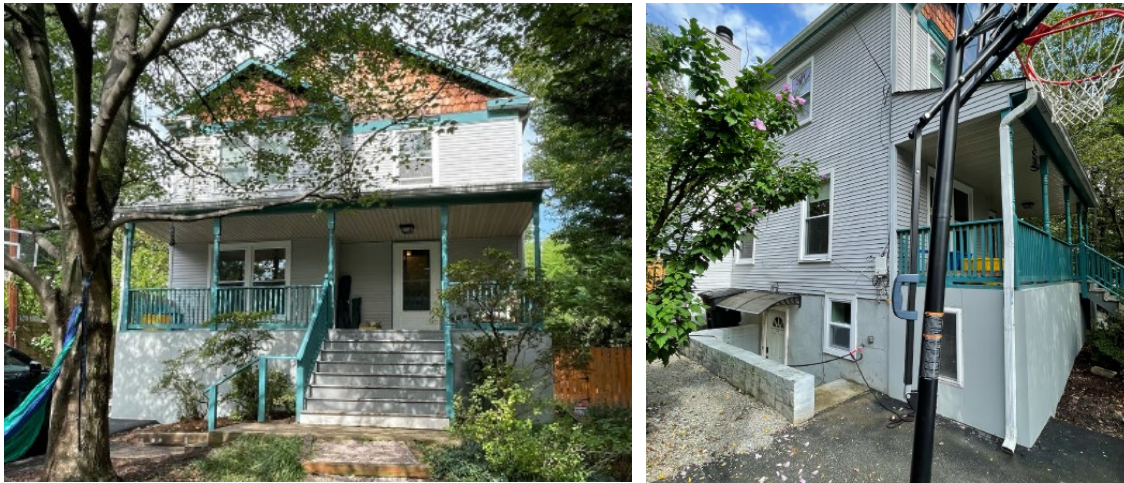
Figure 2: Existing conditions photographs of the front and side elevations.
