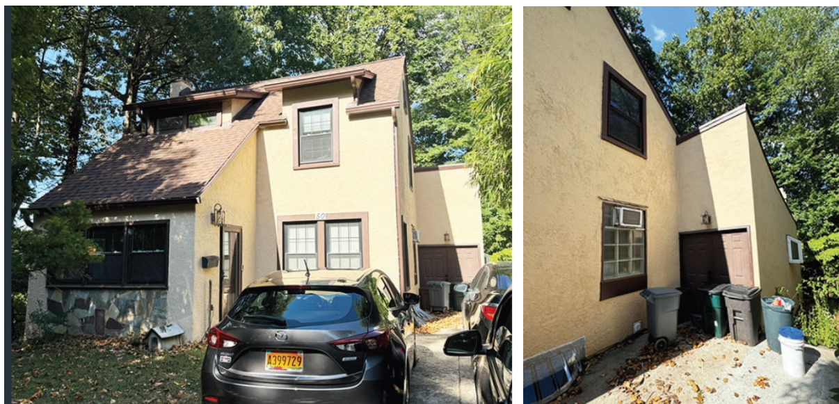
Figure 2: Front and southeast side elevations of the subject property.
