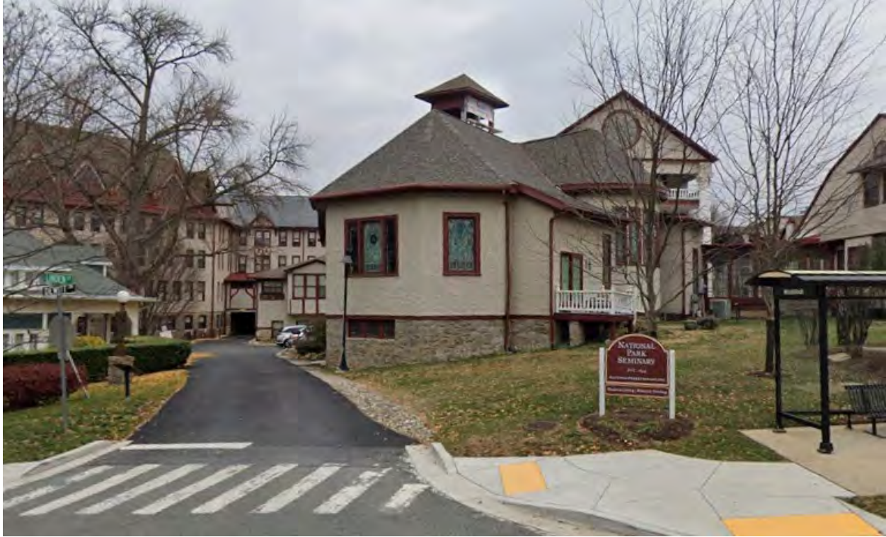
Figure 2: Chapel building from right-of-way along Linden Lane (GoogleMaps, 2025).
