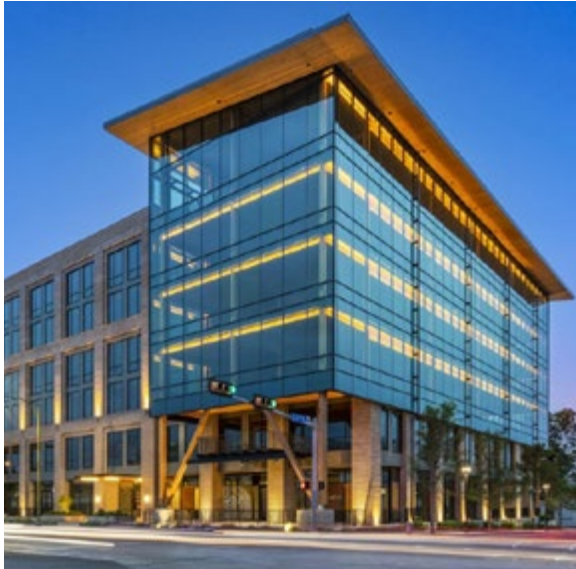
The SOTO building in San Antonio by Lake Flato Architects utilizes a mass timber structural system and includes ground floor commercial retail, office space, and below-grade parking organized around an open courtyard.
