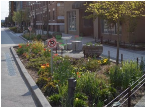
Pervious pavement coupled with planted stormwater facilities can significantly reduce runoff from a site during rain events and reduce flooding risk, a key challenge facing the county that is exacerbated by climate change.
