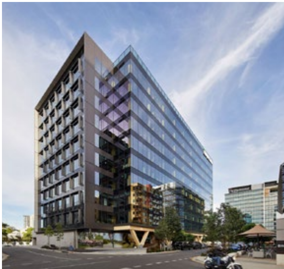
25 King, Brisbane, Australia, is a mass timber tower with a ground floor concrete frame and is a WELL Core Platinum certified structure..
