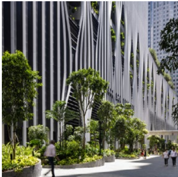
The CapitaSpring Building in Singapore has an exterior façade consisting of vertical elements that are pulled apart to allow glimpses into the green oases blooming from the base, core, and rooftop.
