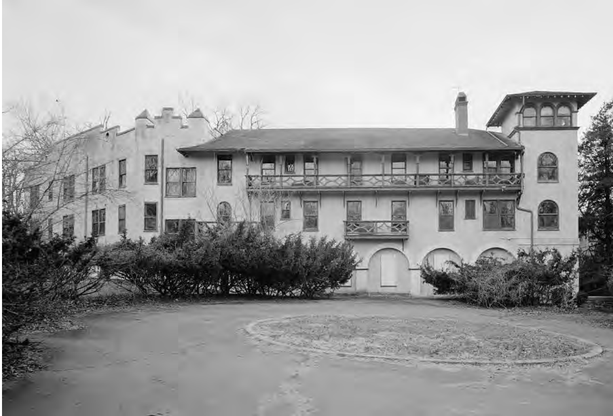
Figure 8: 2001 photographs of the Villa with the since demolished section shown on the left.
