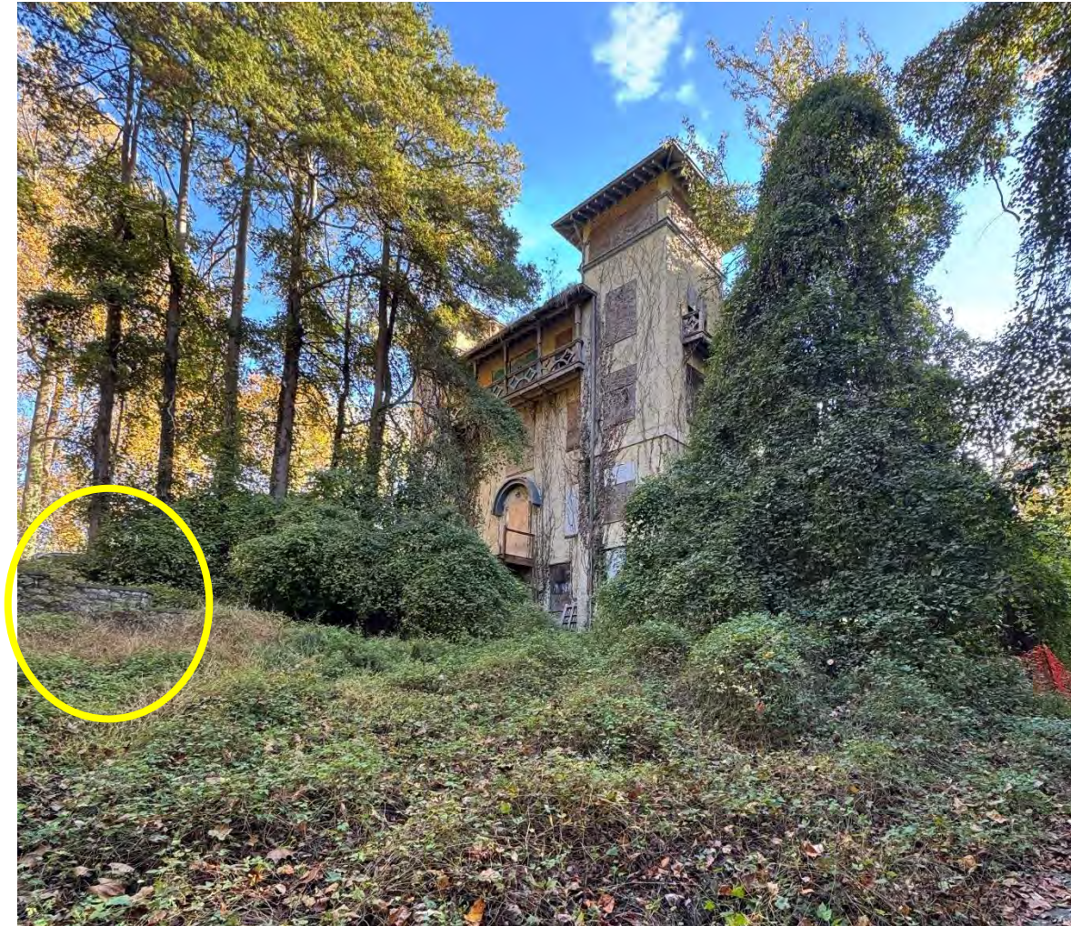
Figure 15: West elevation of the Villa with the stairs shown in Fig. 14 circled in yellow.
