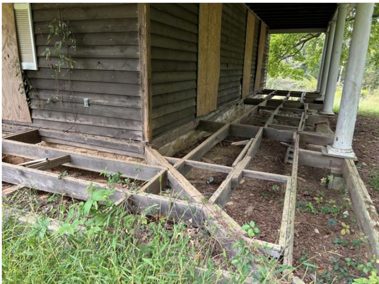
Figure 5: Photograph of the wrap-around porch framing members/structure (September 2025, Historic Preservation Office).
