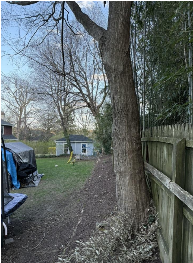
Tree #3, in foreground; Tree #4, seen from a distance and tilting heavily into rear yard of 3924 Baltimore St; and Tree #5, in distance, as seen against garage at 3922 Baltimore St.
