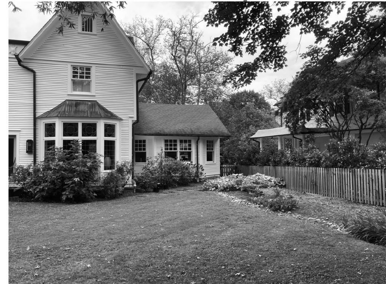
EXISTING CONDITIONS WITH EXISTING FENCE AND GATE
