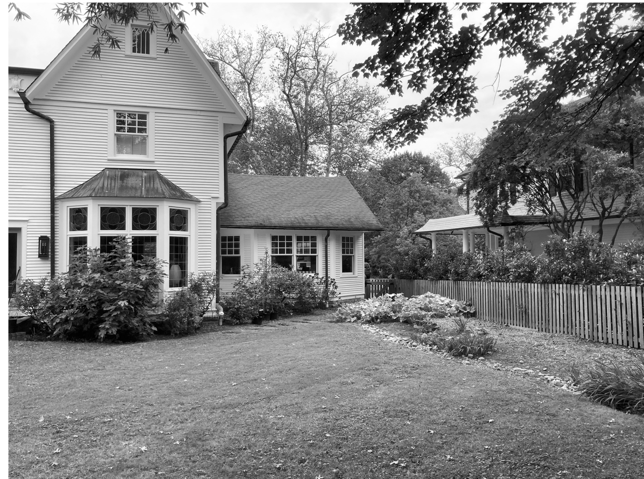
EXISTING CONDITIONS WITH EXISTING FENCE AND GATE
