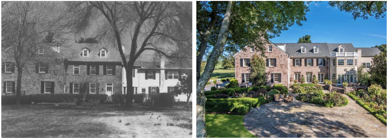
Figure 5: The south elevation of the house in 1988 (left; Carol Humphries) and in 2017 (right; BrightMLS).
