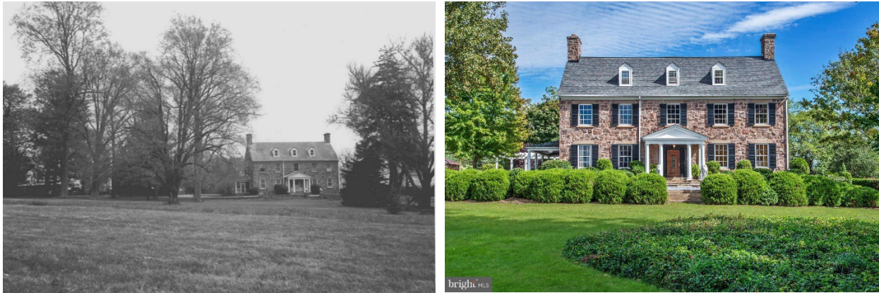
Figure 4: View of front/west elevation of the main house in 1992 (left, Roy Gauzza) and 2017 (right BrightMLS).
