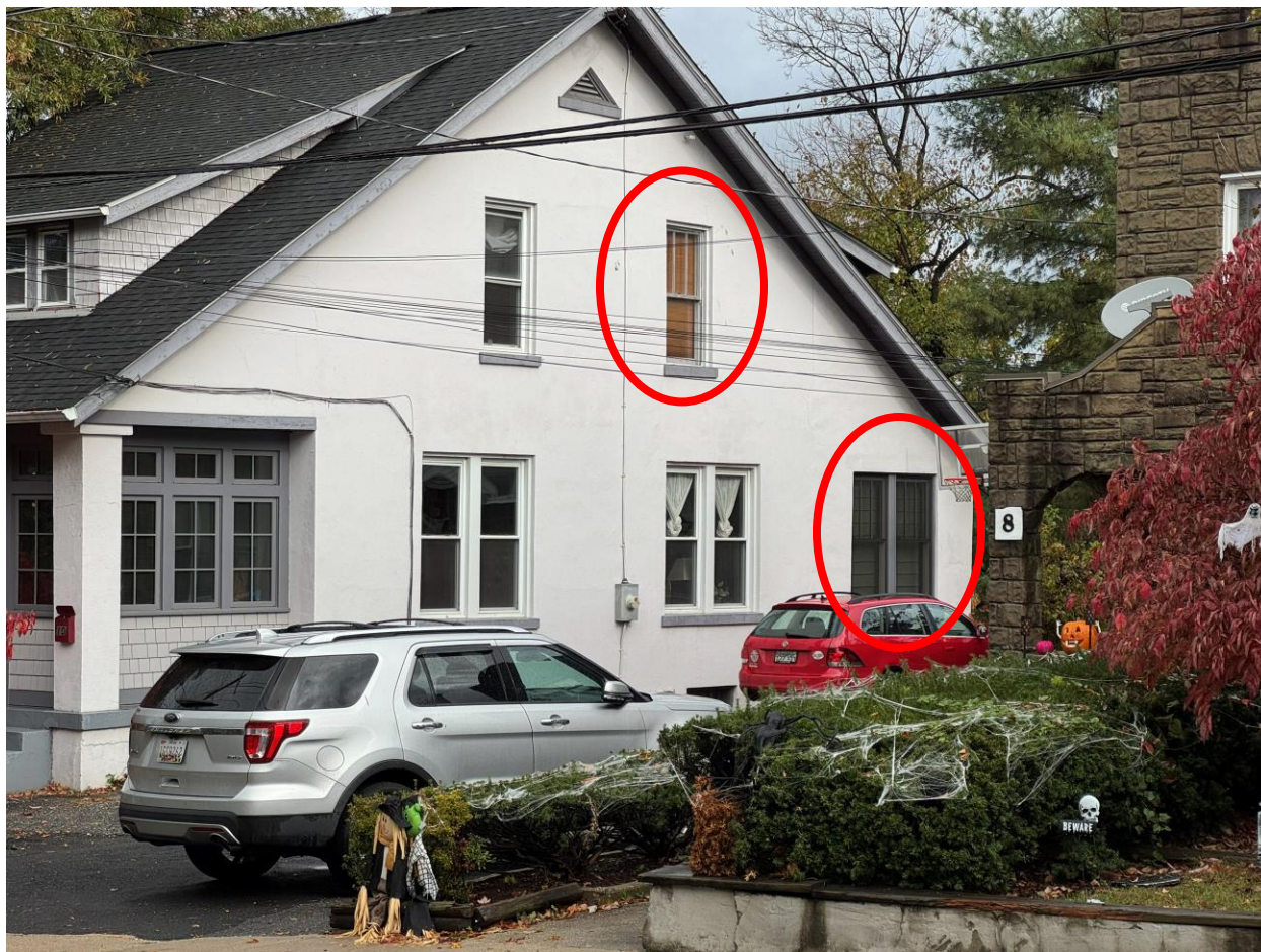
Figure 2: Right side of the subject property. The previously replaced windows are circled in red.
