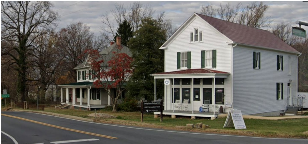
Figure 2: View northwest from the intersection of Darnestown Road and Beallsville Road towards the Darby Store (foreground) and House (November 2024, Google Streetview).
