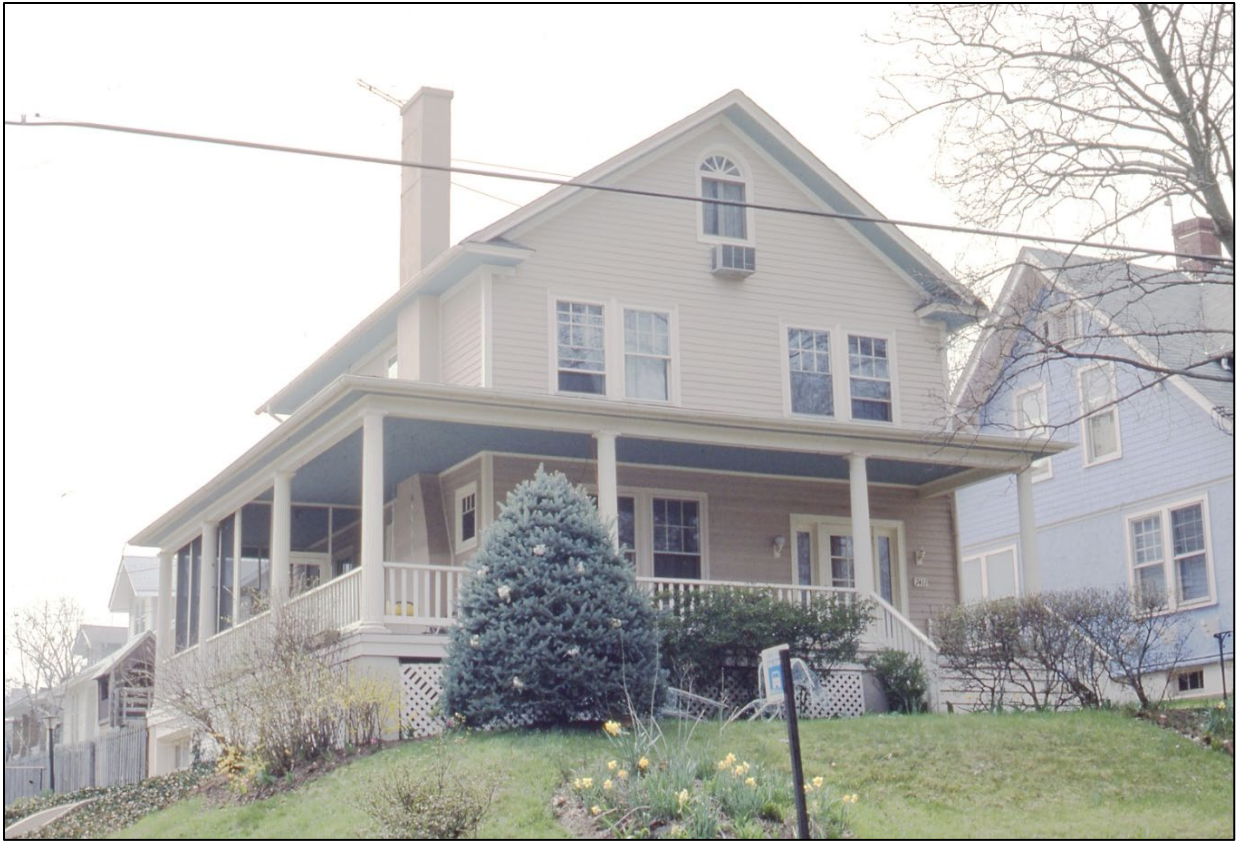
Figure 5: Photo of the subject property c. 1990 (Montgomery County Planning Staff).
