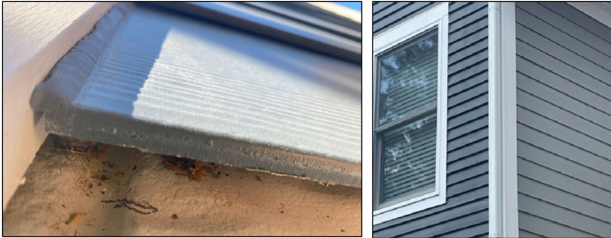
Figure 8: Thickness of the proposed fiber cement siding (left); photo of wood siding on the main house and fiber cement siding on the addition (right; John Sandor, NPS).
