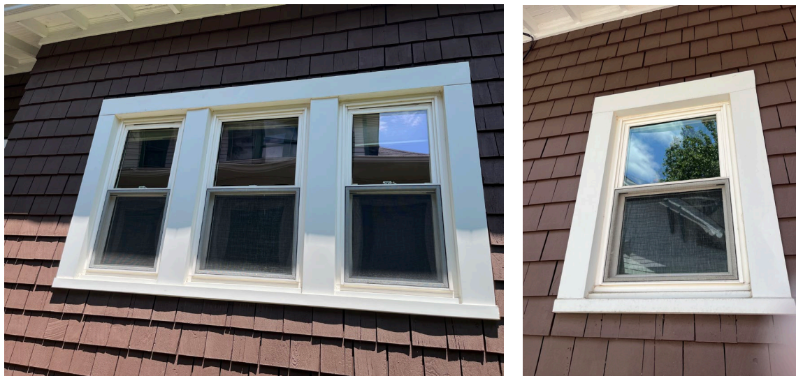
Figure 6: Existing vinyl windows installed (2025). The historic wood trim is capped with vinyl cladding.
