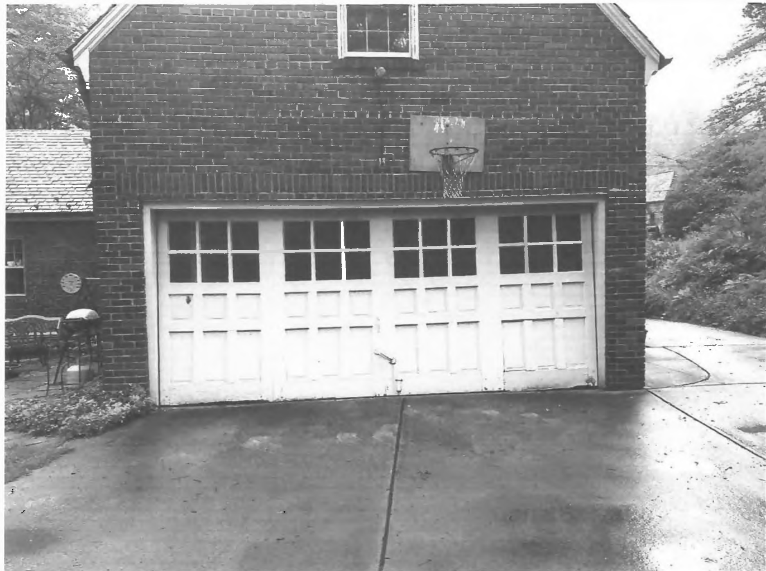
Fig. 2. View of rear-facing garage (essentially south-facing), showing original manually operated overhead garage double door in closed position.
