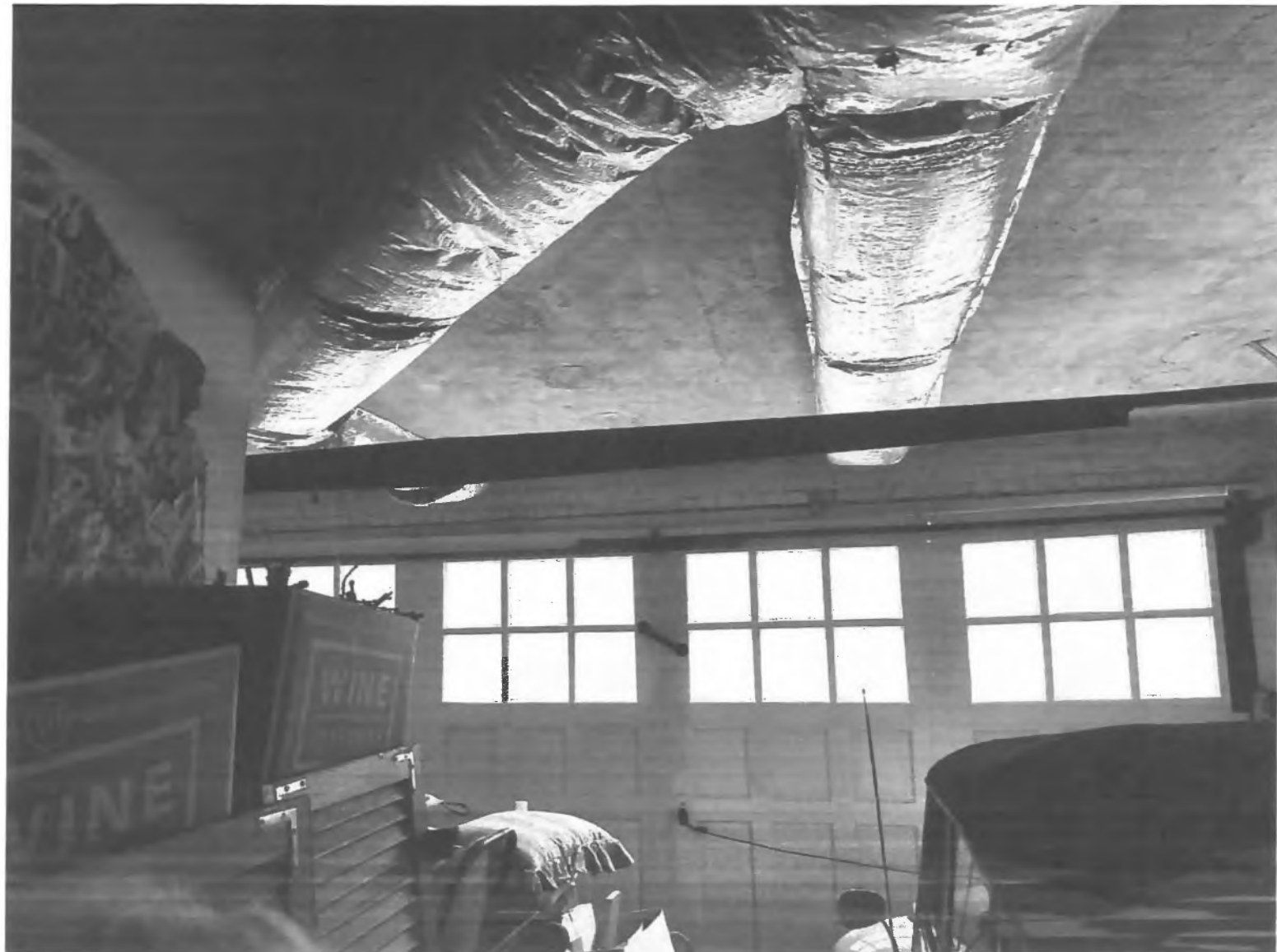
Fig. 4. Interior view of garage (essentially south-facing), showing HVAC air ducts mounted on garage ceiling.
