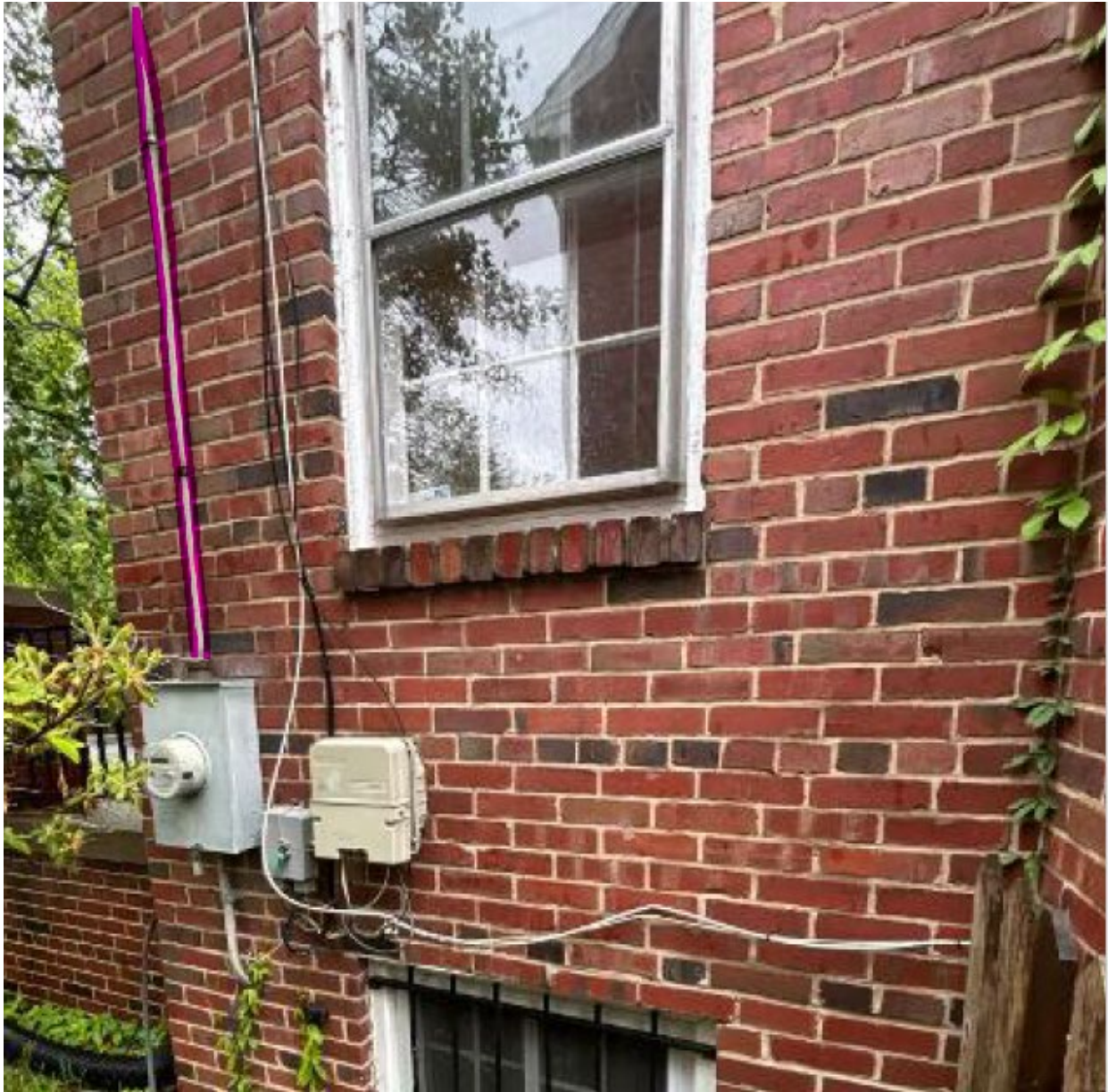
Utility Meter after Install. To run along side the meter/conduit and along the roof ridge to the Array.
