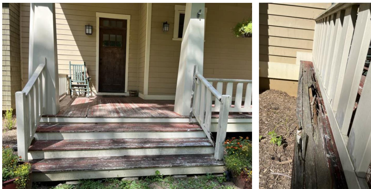
Figure 4: Existing conditions of the porch decking to be replaced.
