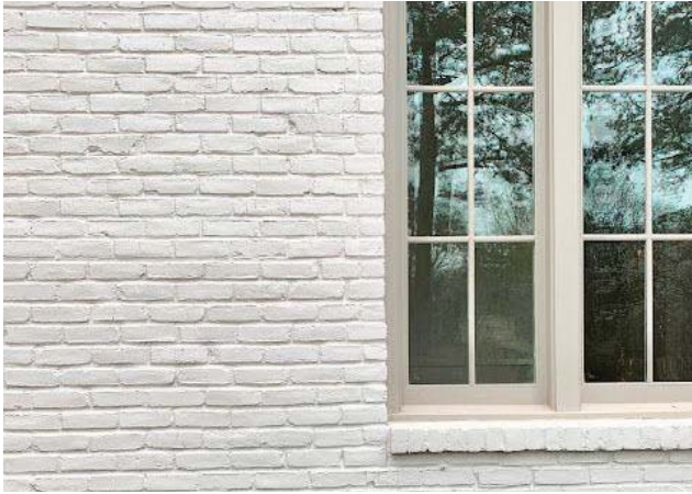
PAINTED BRICK New brick to match existing in size, color and texture. New and existing brick to get painted.
