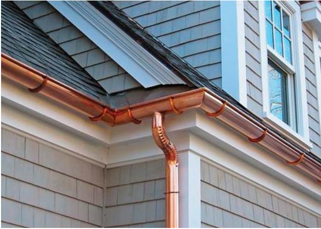
METAL GUTTERS & DOWNSPOUTS 6" copper half round and 4" full round downspouts. Run all downspouts to cast iron sleeves connected to underground drain pipes.
