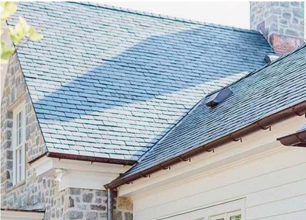
SLATE ROOF Slate shingles to match existing. Contractor to provide samples to confirm new slate size, color and texture. Salvage and re-use slate where appropriate.
