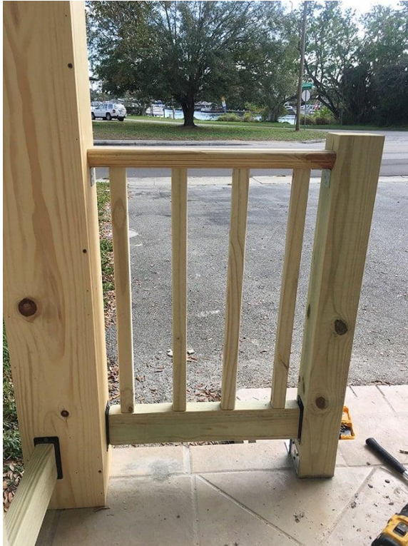
Figure 5: This railing has the pickets installed between the top and bottom rails.
