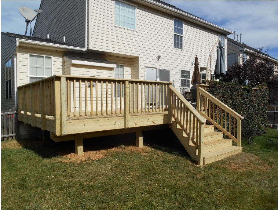
Figure 4: A sweeper-style railing installed by the contractor.
