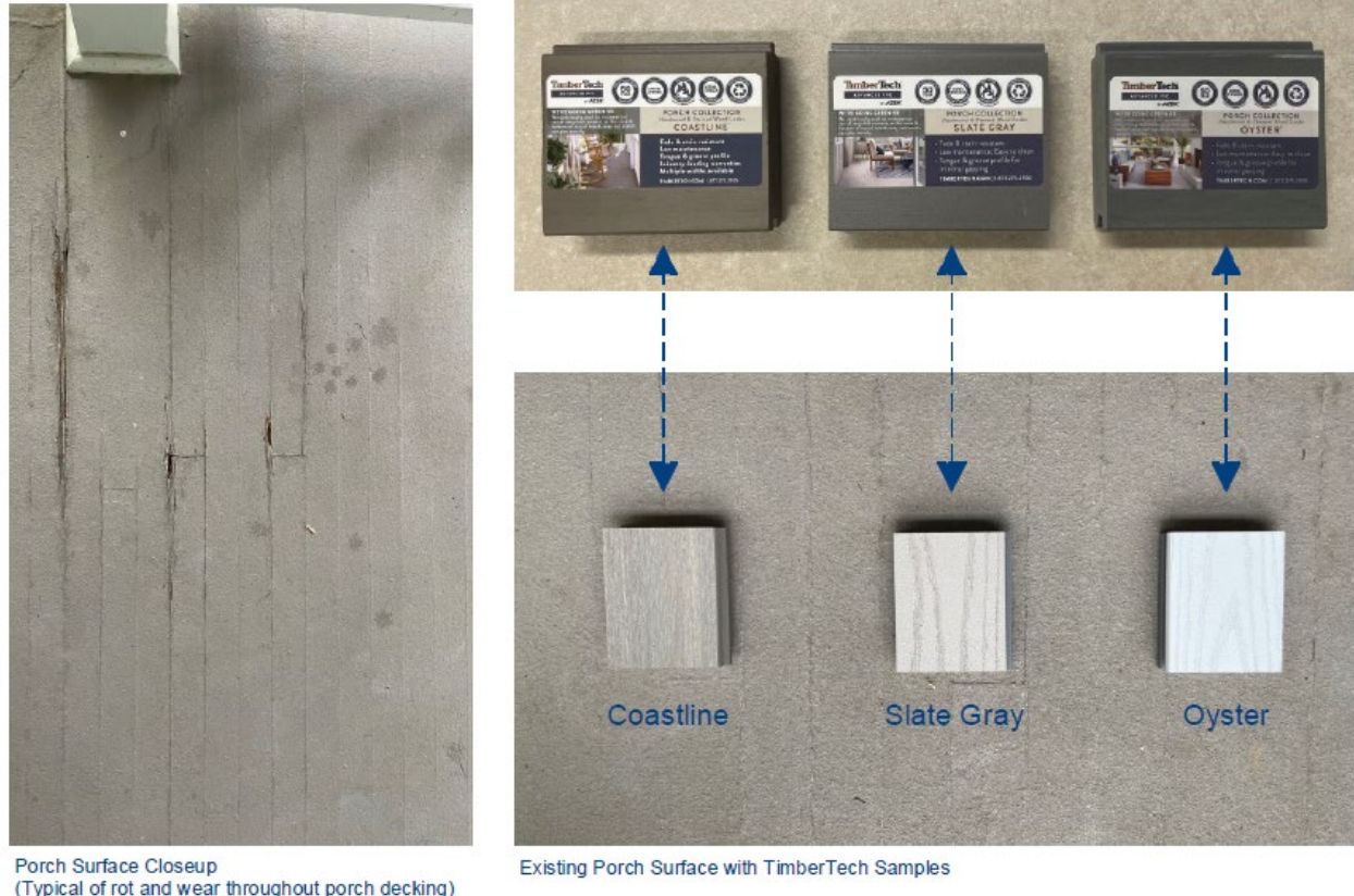
Figure 7: Existing and proposed porch floor materials.
