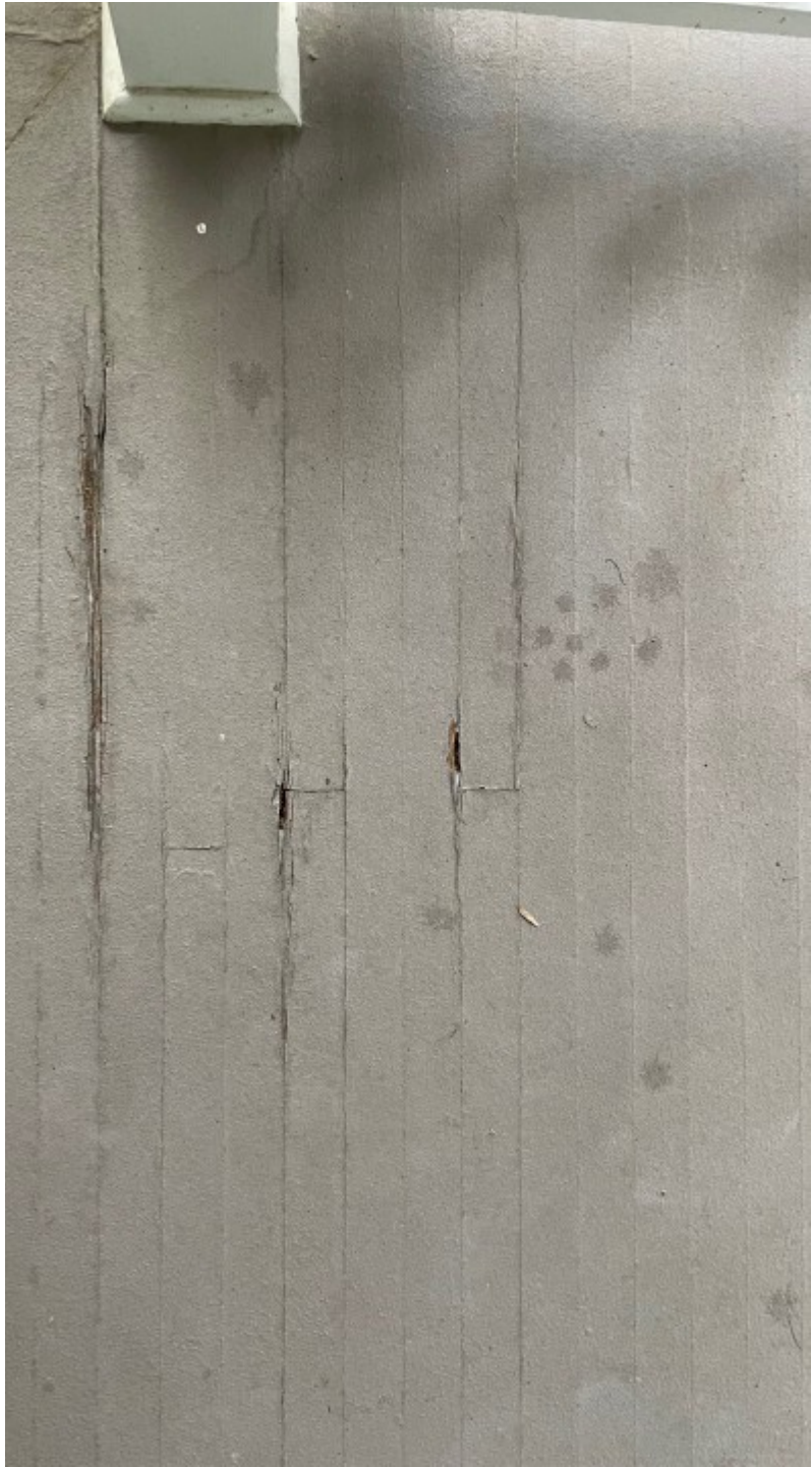
Porch Surface Closeup (Typical of rot and wear throughout porch decking)
